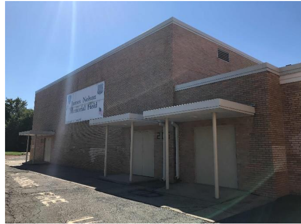
Side of Building
