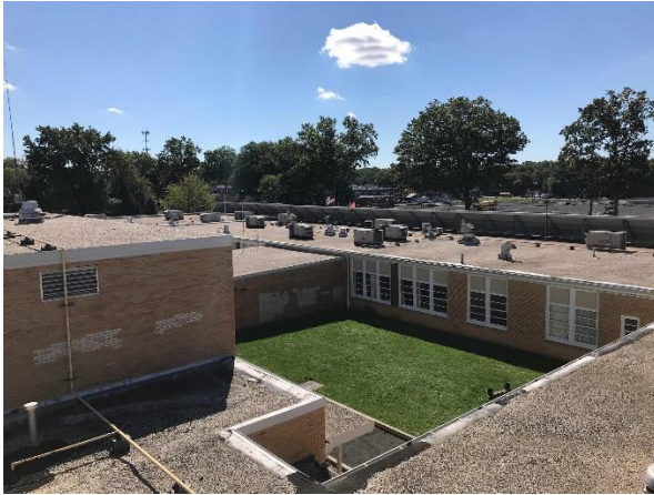
Building Roof Top
