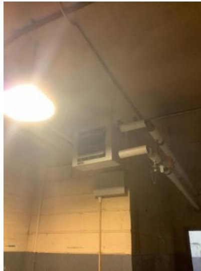
Basement Storage Room – Unit Heater
