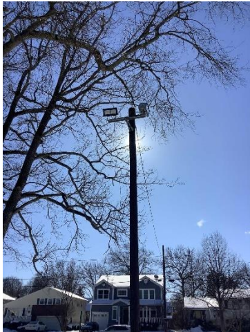
Exterior pole mounted LED fixture
