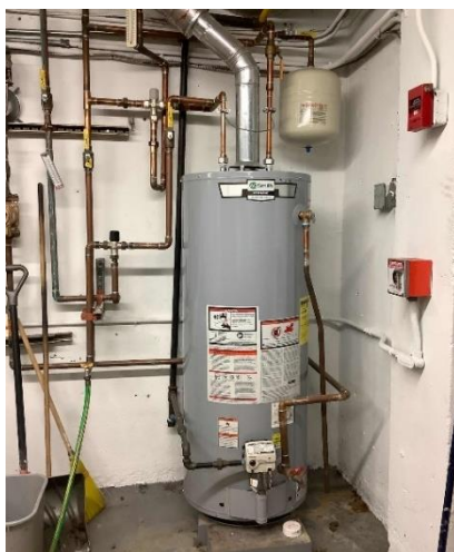
Gas Fired DHW Heater
