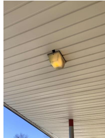
Exterior surface Mounted fixture
