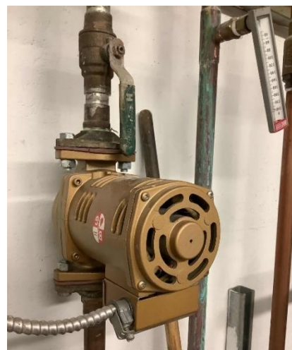
DHW Recirculation Pump
