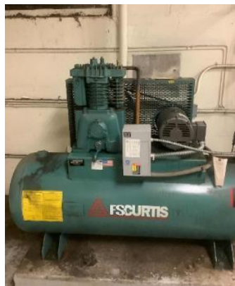
Air compressor for pneumatic valves
