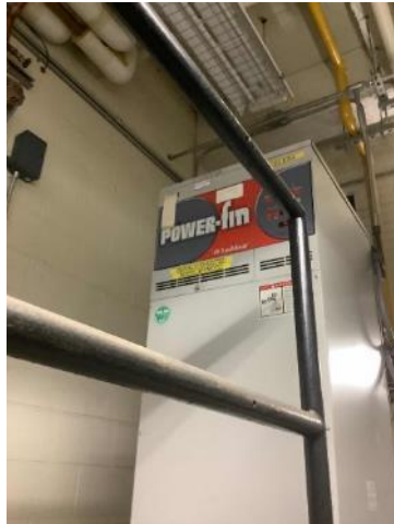
Gas fired DHW heater
