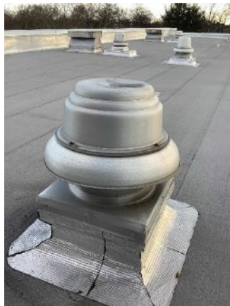
Exhaust fans on the roof
