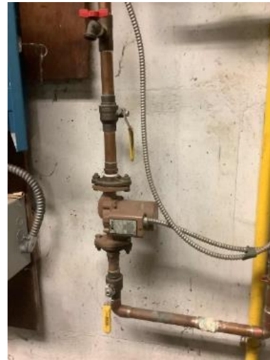
DHW Recirculation Pump
