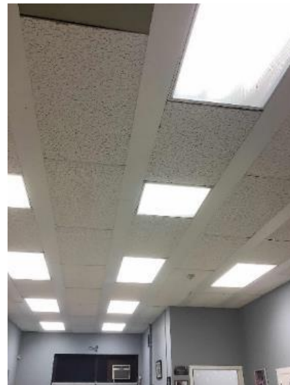
Office 4-foot T8 Prismatic fixtures
