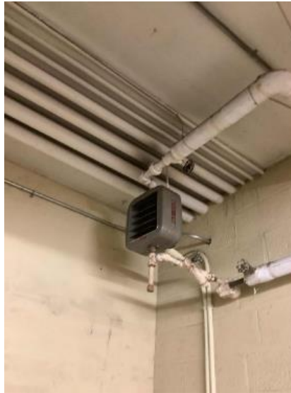
Boiler room – Unit Heater
