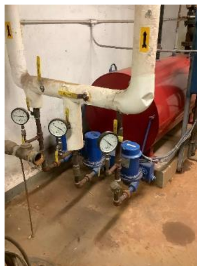
Feed Water Tank and Pumps
