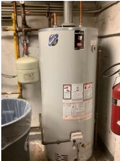
Gas fired DHW Heater
