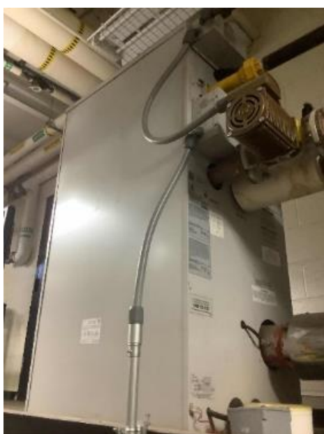
Gas fired DHW heater
