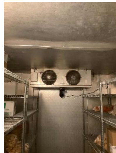
Walk-in cooler evaporator fan
