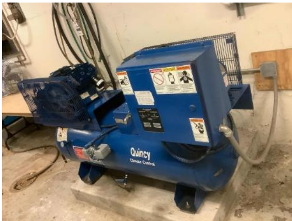
Air compressor for pneumatic valves
