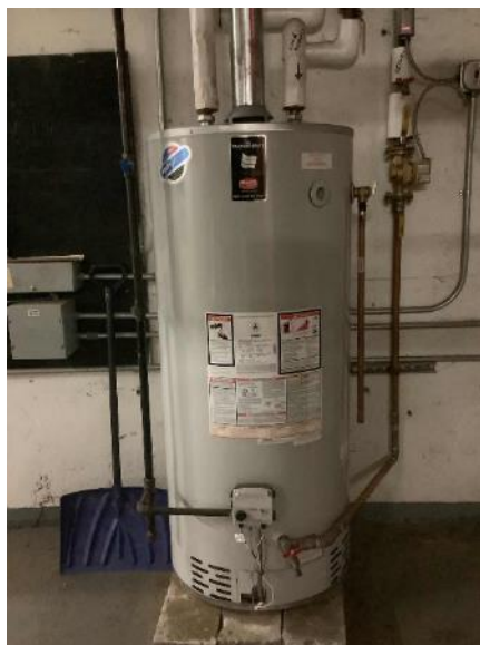
Gas Fired DHW heater
