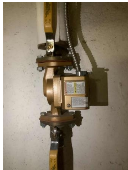
DHW recirculation pump
