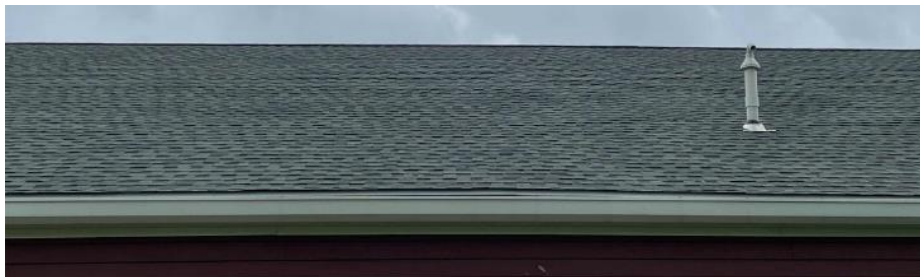
Pitched Asphalt Shingle Roof
