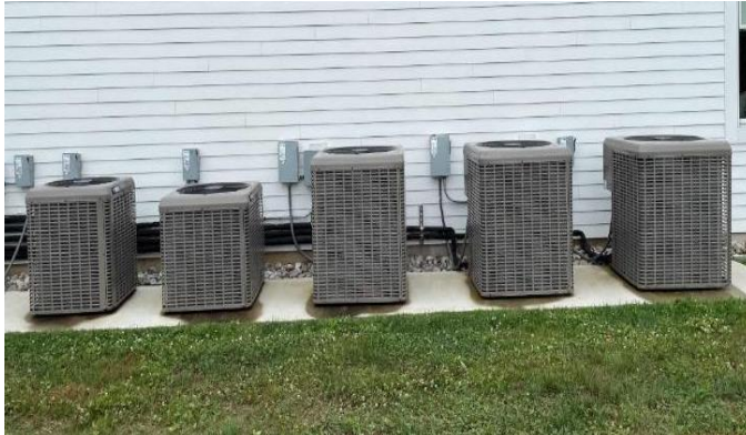
Exterior Condensing Units
