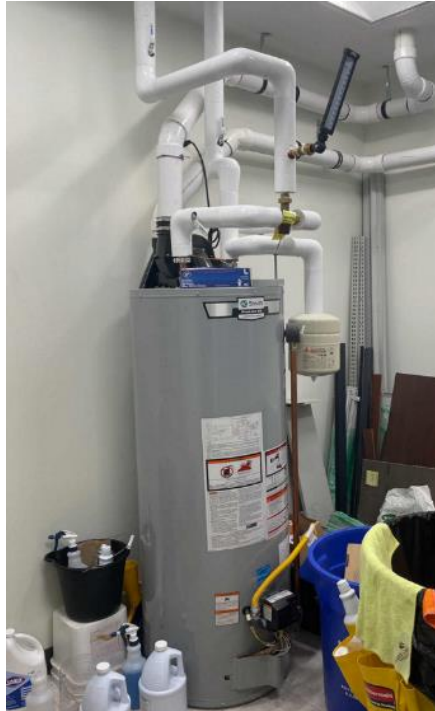
Gas Fired DHW Tank
