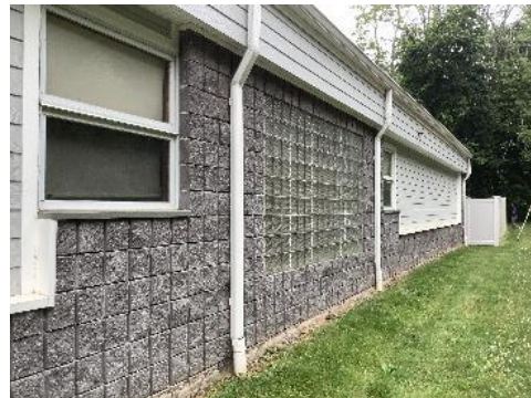
Roadside View of the Building Siding
