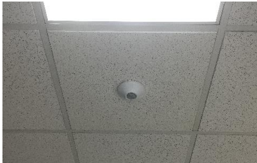
Ceiling-Mounted Occupancy Sensor
