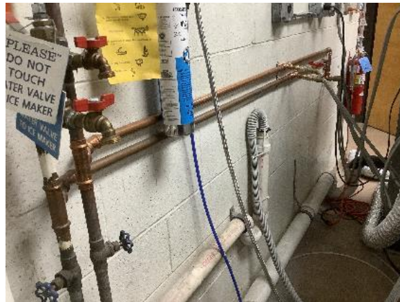
Domestic Hot Water Clothes Washer Supply
