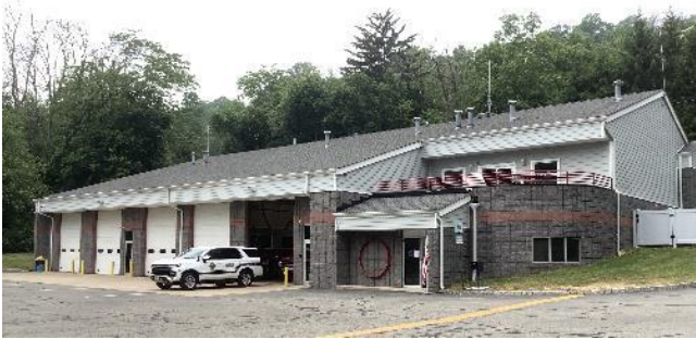
Garage Doors and Parking Lot View of Building
