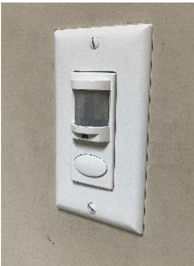
Wall-Mounted Occupancy Sensor
