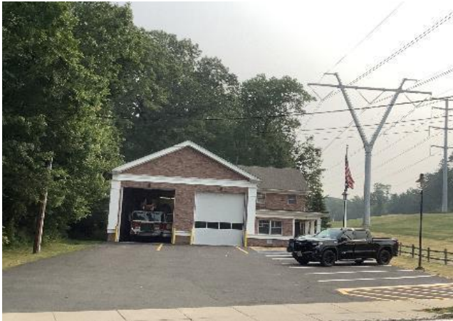
Front of Building
