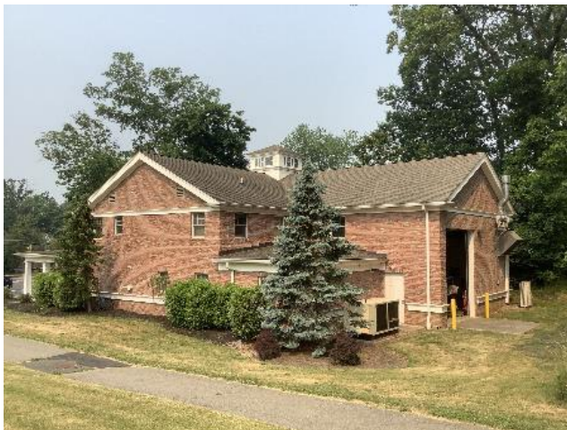
Side View of Building and Roof
