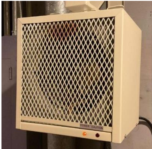
DePaul High School: Electric Resistance Heater & Dial Thermostat
