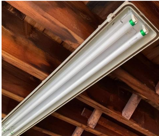
Maintenance Garage: Linear Fluorescent T8 Lamps
