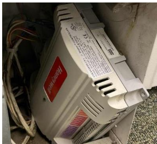
DePaul High School: Unit Ventilator Honeywell Controller
