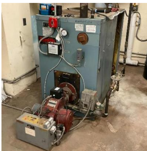
DePaul High School: HHW Boiler & HHW Supply Pumps
