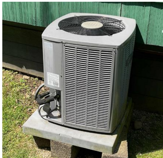
Art Annex: Split AC Condensing Unit
