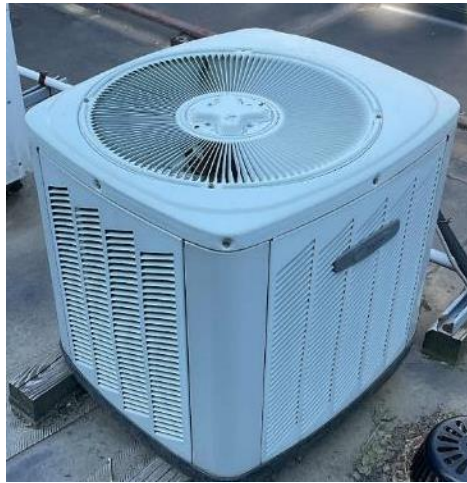
DePaul High School: Roof Mounted AC Condensing Unit
