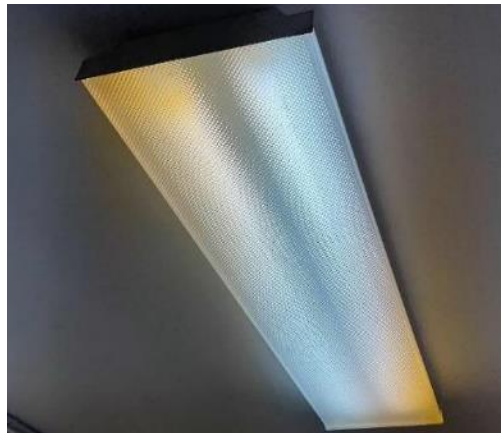
Snack Stand: Interior Linear Fluorescent Lights
