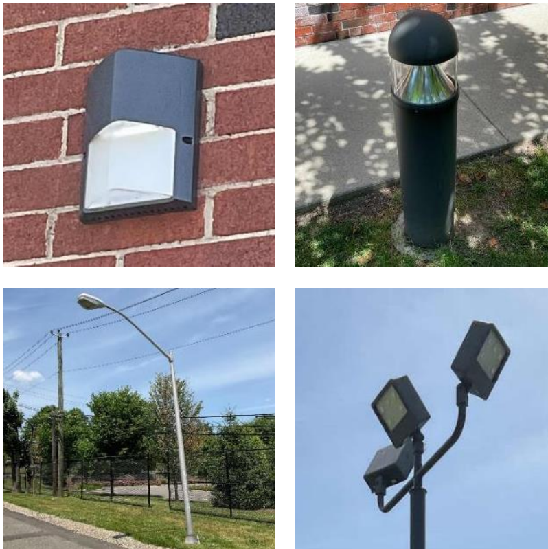
DePaul High School: LED Wall Pack, LED Bollard, and LED Pole Mounted Fixtures
