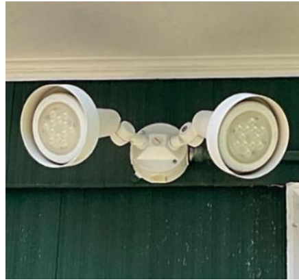
Art Annex: Exterior Socketed LED Lamps w/ Photocell Control
