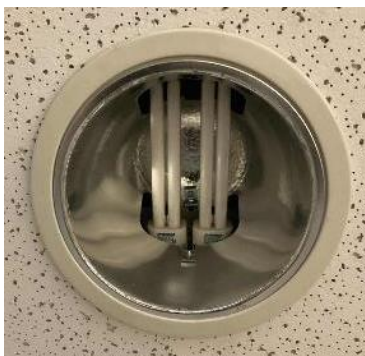
DePaul High School: Recessed Can Plug-In CFL Lamps, A19 Incandescent, and Downlight Recessed LED Fixture
