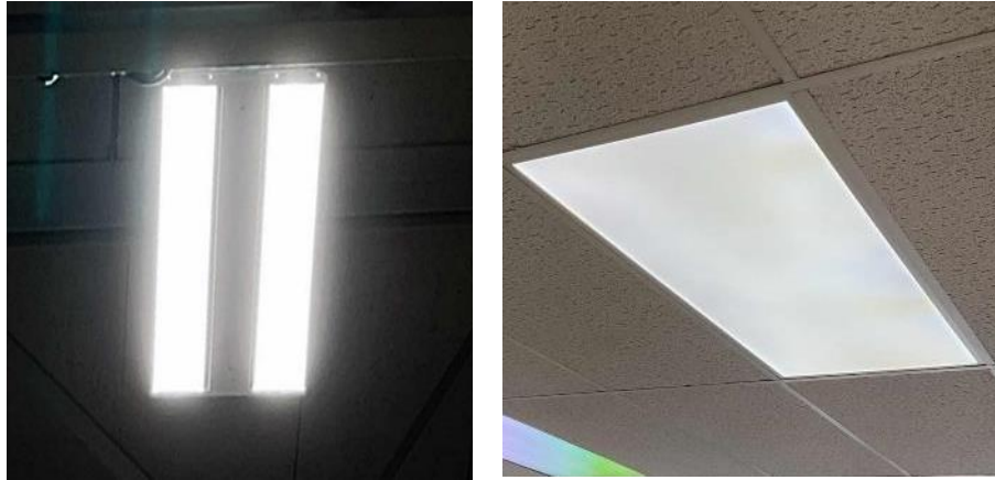
DePaul High School: Gym LED High Bay Fixture and LED 2x5 Ambient Panel
