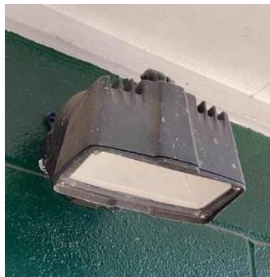
Snack Stand: LED Wall Pack and LED Field Lighting
