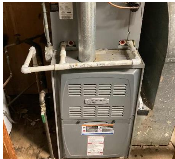
Art Annex: Forced Hot Air Furnace
