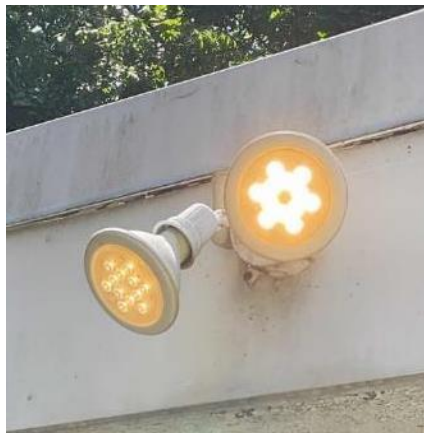
Maintenance Garage: LED PAR38 Lamps and LED A19 Lamp
