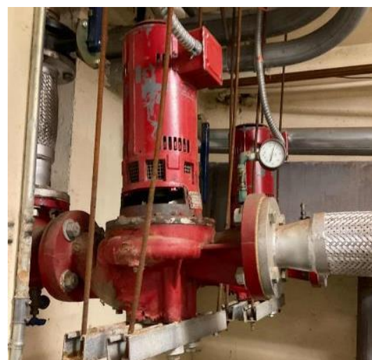
DePaul High School: HHW Boiler & HHW Supply Pumps
