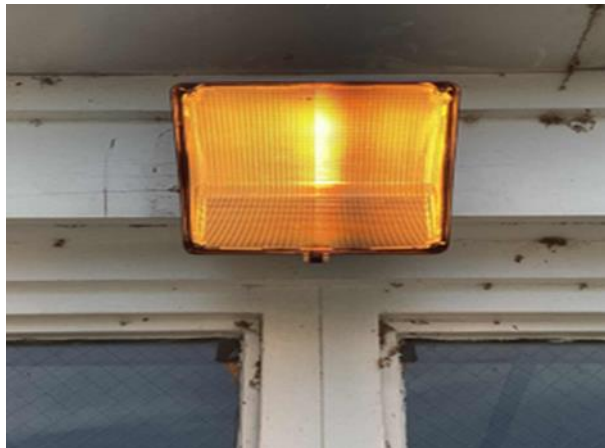
High-Pressure Sodium Wall Pack
