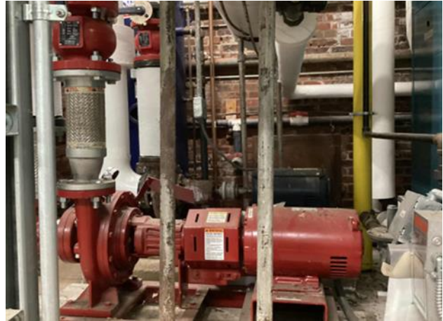
Heat and Hot Water Pumps
