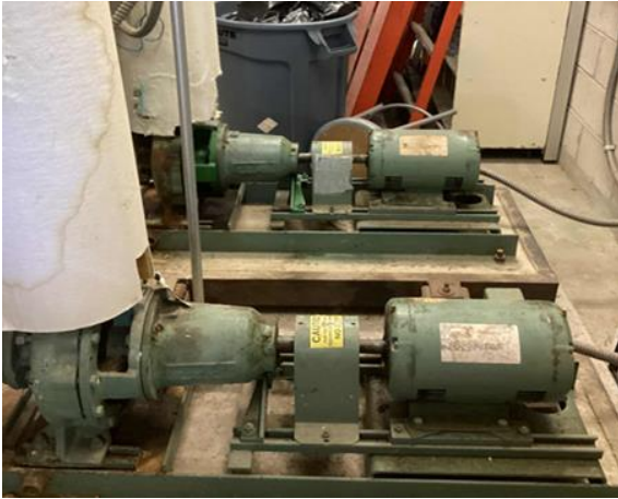
Heat and Hot Water Pumps
