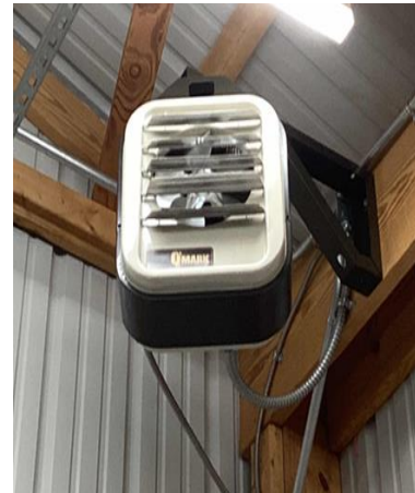
Suspended Electric Resistance Heater
