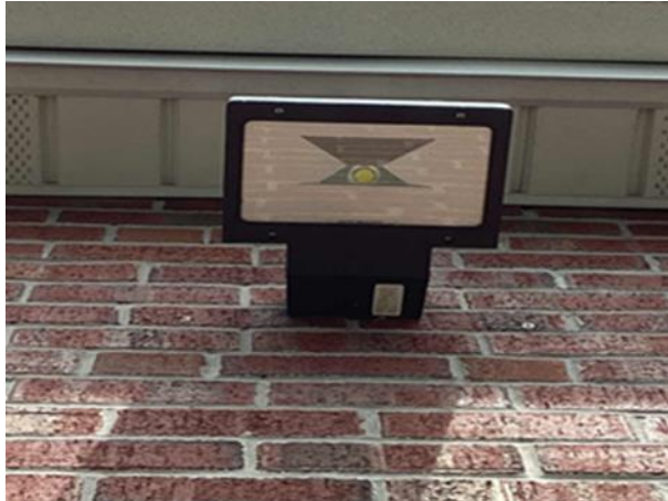
LED Flood Fixture
