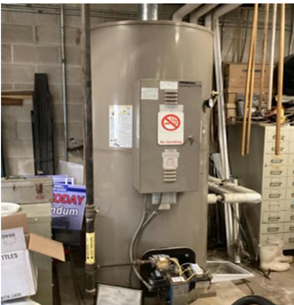
Gas-fired Water Heater
