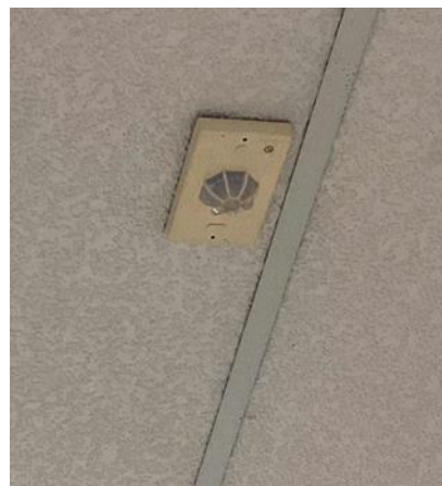
Ceiling-Mounted Occupancy Sensors
