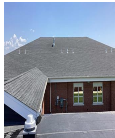
Pitched Roof with Asphalt Shingles
