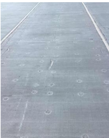
Flat Roof with Black Rubber Membrane
