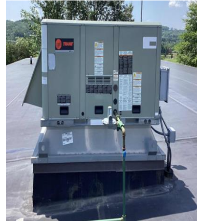
Roof Top Package Unit
