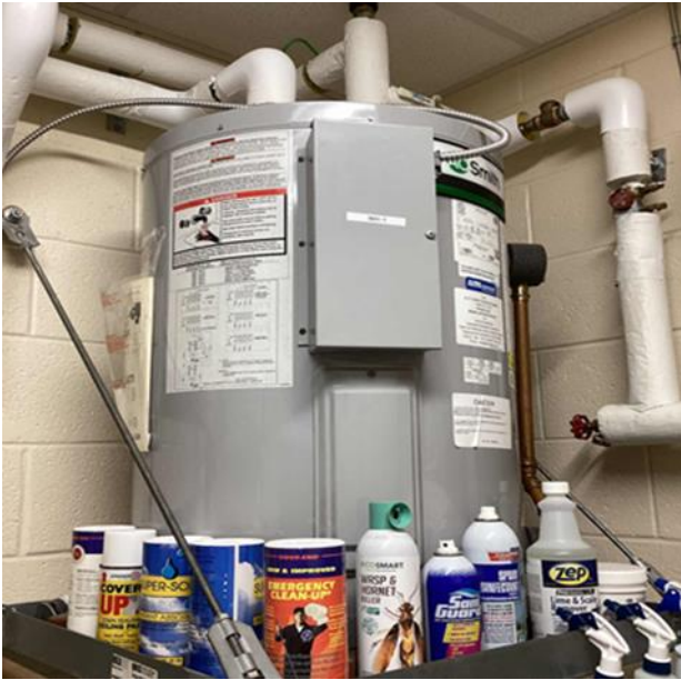
Electric Water Heater
