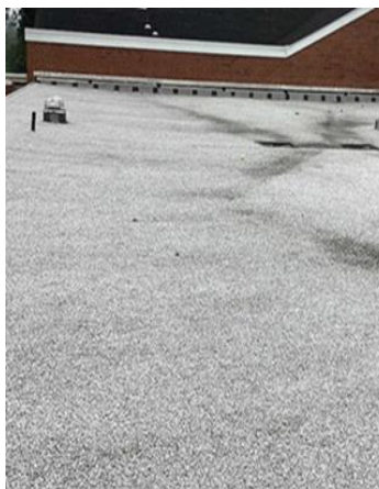
Flat Roof with Gravel Finish
