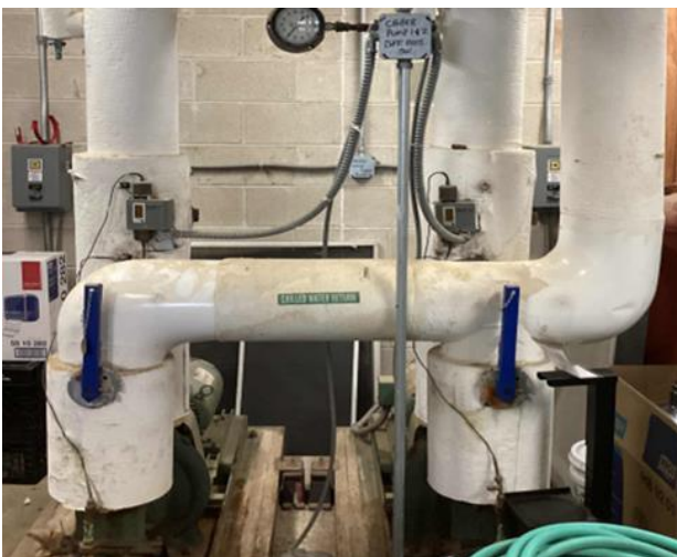
Chilled Water Pumps and Tag
