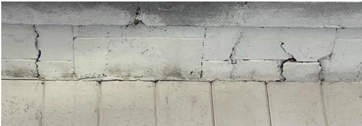
Damaged KVSP Envelope Section
