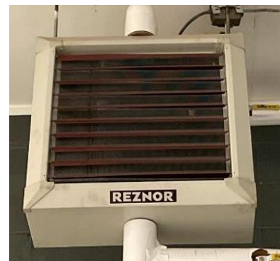
Hydronic Unit Heater
