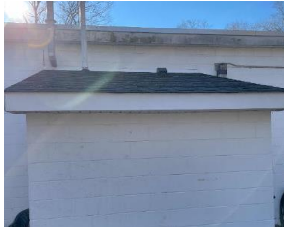
Pitched Asphalt Single Roof
