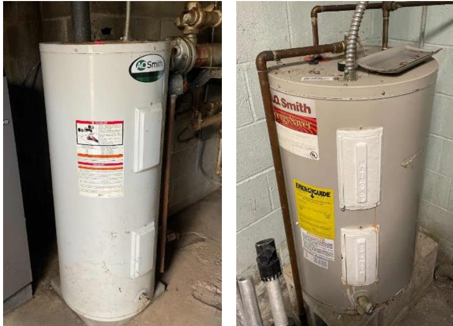
Aeroflex A.O. Smith DHW Tanks
