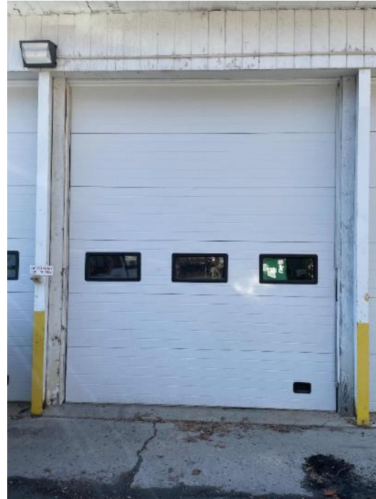
Overhead Garage Door with Single Pane Glass Windows
