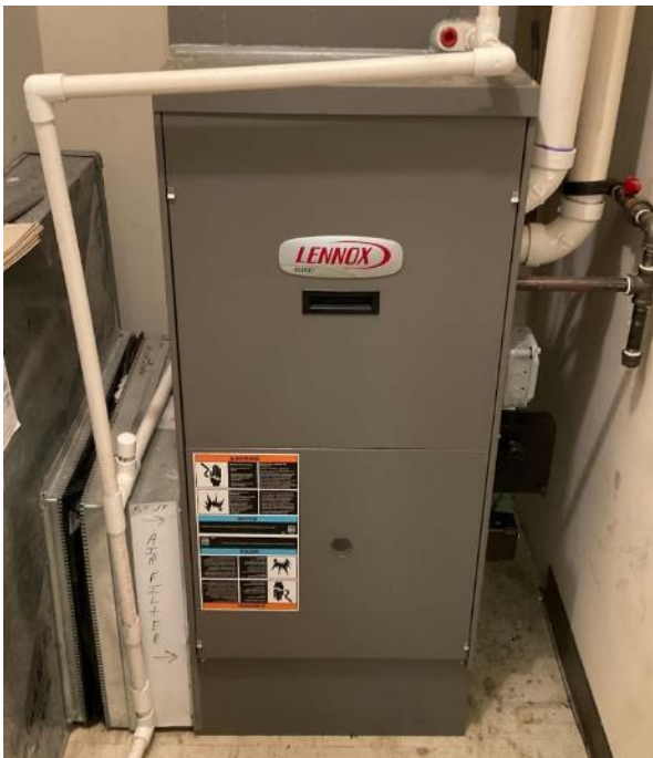
AHU and Forced Gas Furnace
