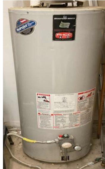
Storage Tank Water Heater
