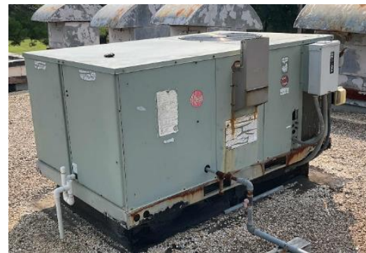
Package Unit on Scout Building Roof
