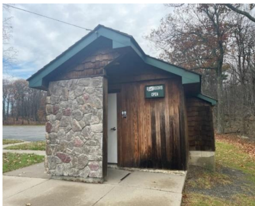
Restroom Envelope with Stone Façade AND Wood Siding
