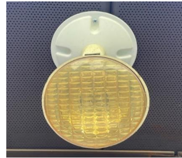
Bathhouse: Exterior Halogen & LED Wall Pack
