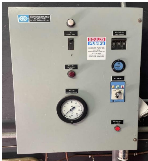
Well Water Supply Pump Control Box
