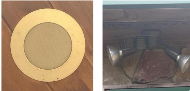
Restroom: LED Downlight Recessed Fixture & LED PAR Lamps
