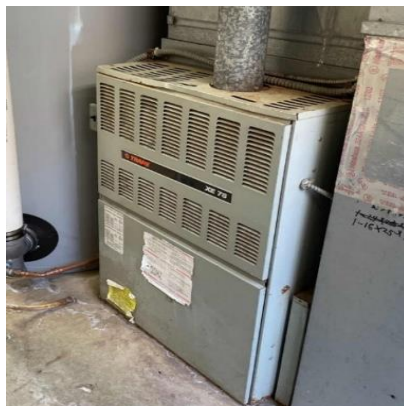
Bathhouse: Propane Fired Furnace
