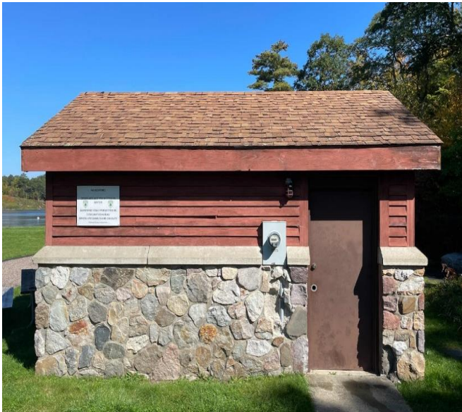
Pumphouse Envelope with Stone Facade and Wood Siding
