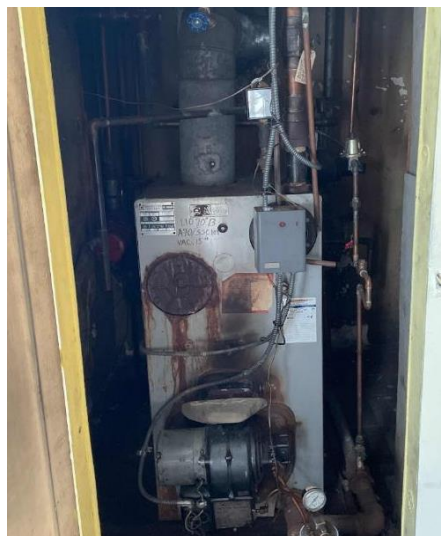
Non-Condensing HHW Boiler
