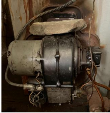
Oil Combustion Burner
