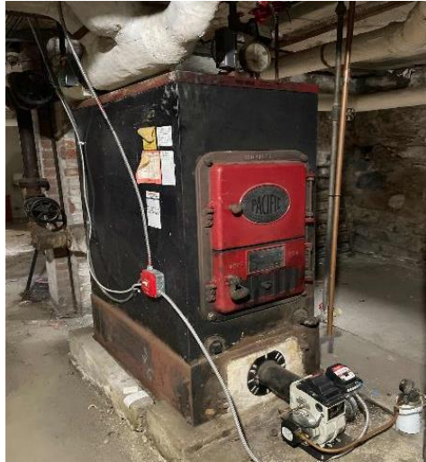
Non-Condensing HHW Oil Boiler
