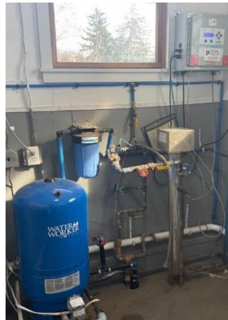
Well Pump Pressure Tanks with UV Filter System
