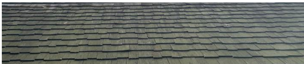
Sawmill Restroom: Cedar Shingle Roof
