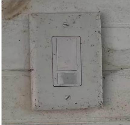
Wall Mounted Occupancy Sensor
