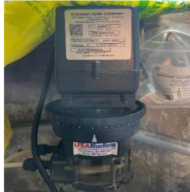
Sawmill Pumphouse: Chlorine Pump
