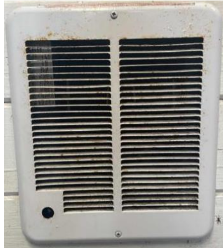
Sawmill Restrooms: Electric Resistance Heater W/ Removed Dial Control
