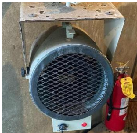
Electric Resistance Heater
