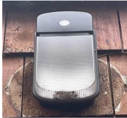
LED Wall Pack W/ Integrated Photocell
