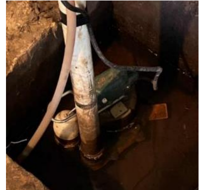
Sawmill Pumphouse: Sump Pump
