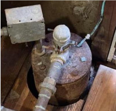
Sawmill Pumphouse: Well Water Supply Pump
