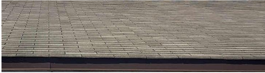
Asphalt Shingle Roof
