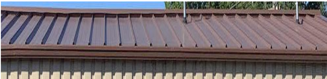
New Garage Standing Seam Metal Roof
