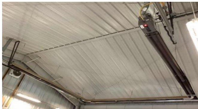
Suspended Propane Heater
