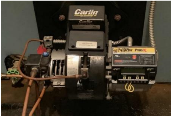
Office-Shop Boiler Combustion Air Fan
