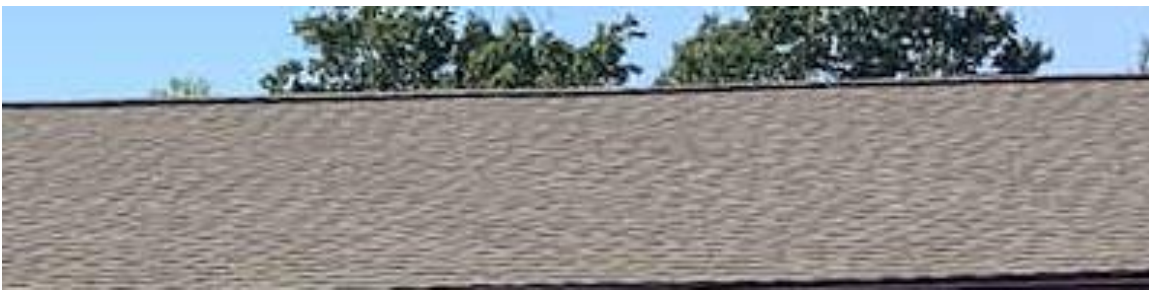
Office-Shop Asphalt Shingle Roof
