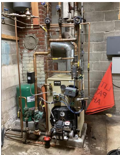
Hot Water Boiler
