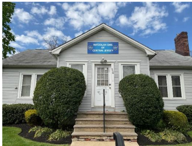
Pitched Roof with Asphalt Shingles
