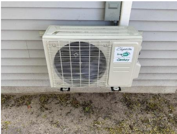
Split-System Air-Source Heat Pumps in Storage Shed
