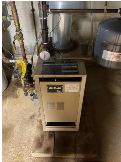
Weil McLain Heating Hot Water Boiler
