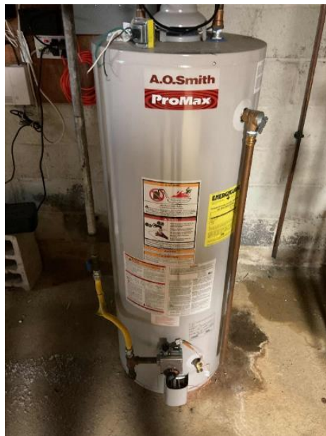
Main Building Storage Tank Natural Gas Water Heater
