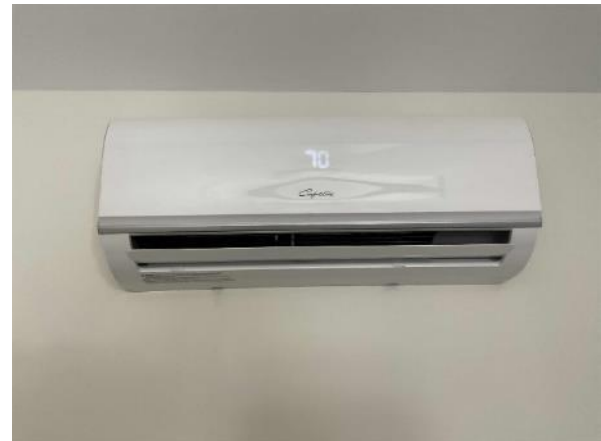
Split-System Air-Source Heat Pumps in Storage Shed
