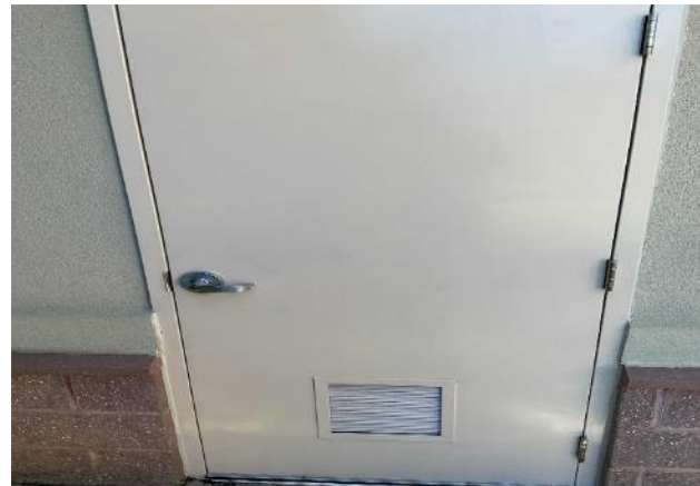
Typical Exterior Door
