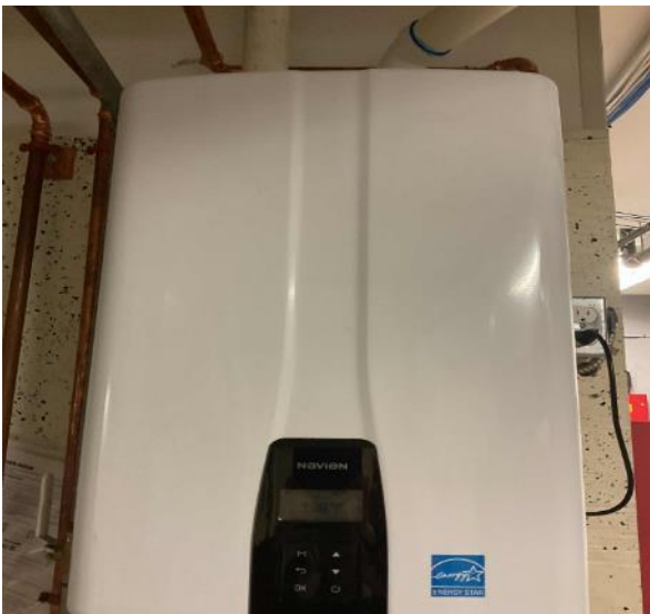
Navien Natural Gas Tankless Water Heater
