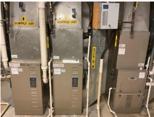
Carrier Gas-Fired Furnaces
