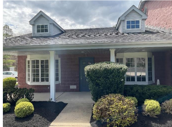
Pitched Roof with Asphalt Shingles
