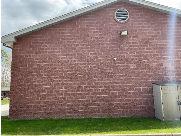
Typical Exterior Walls
