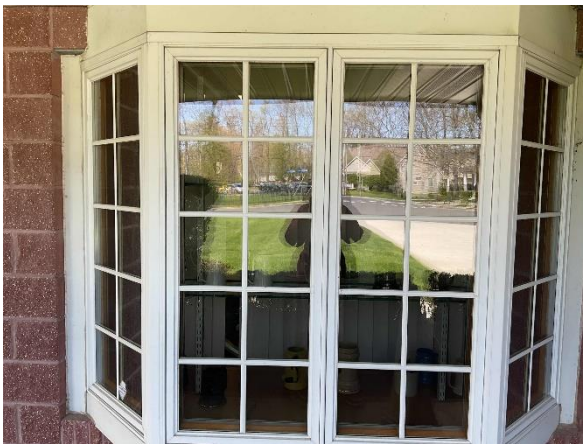
Typical Facility Windows
