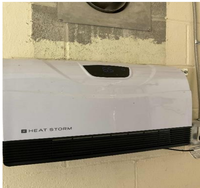
Electric Resistance Unit Heater
