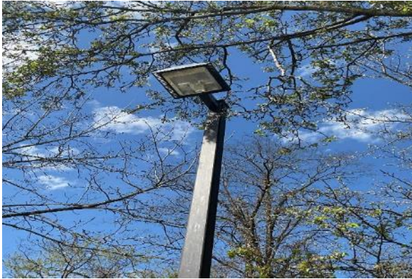
Pole Mounted Parking Lot LED Lighting
