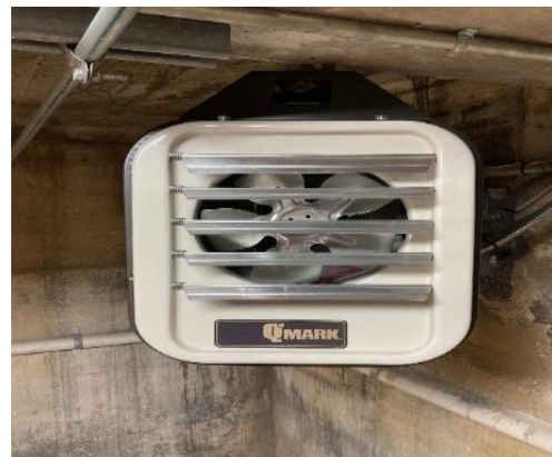
QMark Unit Heater in Basement
