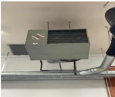
Modine Unit Heater in Garage
