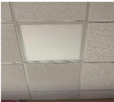
LED 2-foot x 2-foot Fixture
