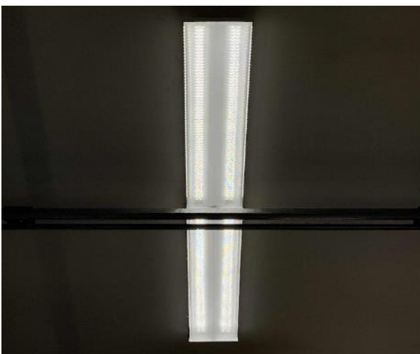
LED Linear Strips in Garage
