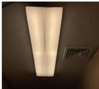
LED 2-foot x 4-foot Light Panels
