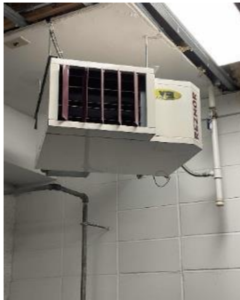
Reznor Natural Gas Unit Heater
