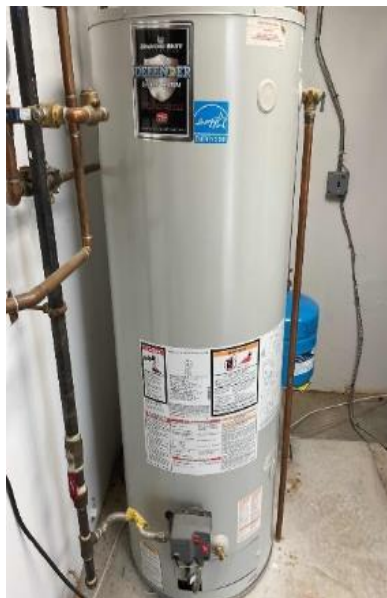
Bradford White Natural Gas Storage Tank Water Heater
