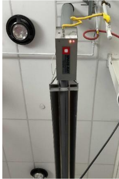
Space Ray Infrared Heaters Installed in Garage
