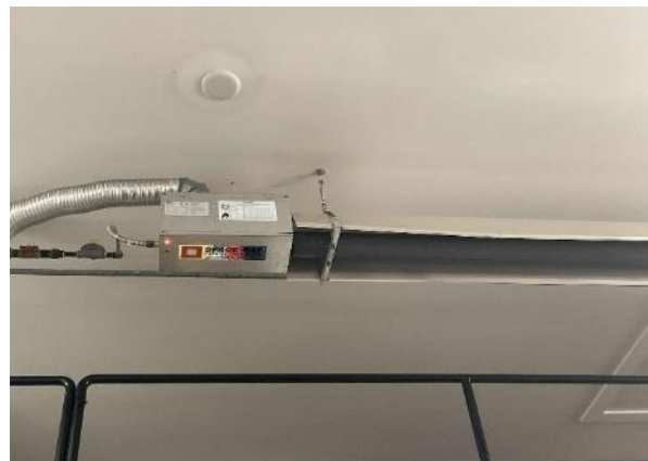
Gas-Fired Infrared Heaters
