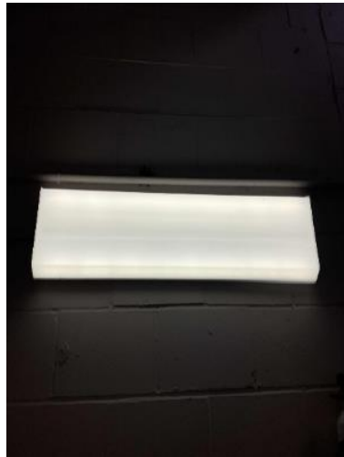
LED 2-foot x 2-foot Light Panel Fixture
