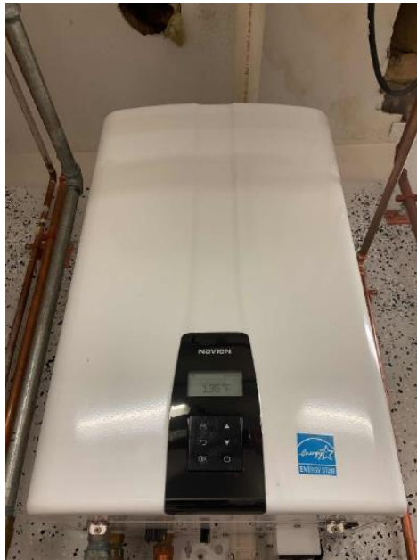
Navien Gas-Fired Tankless Water Heater
