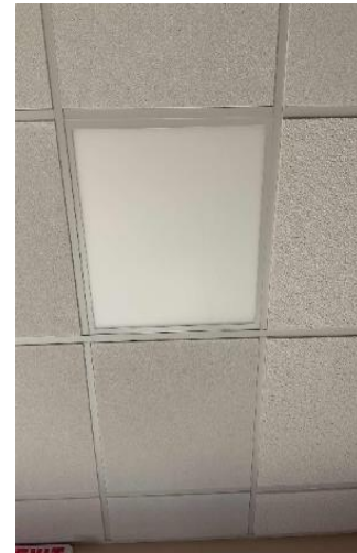
T8 Equivalent LED Lamp Fixture
