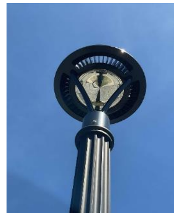
LED Pole Mounted Exterior Parking Lot Lights
