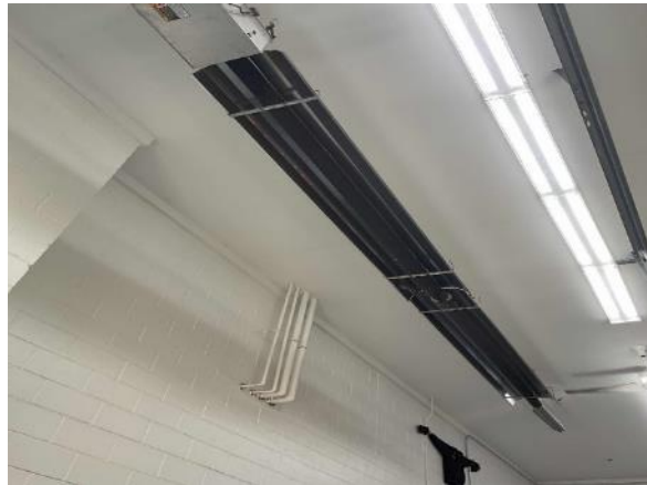
Reznor Infrared Heater in Garage
