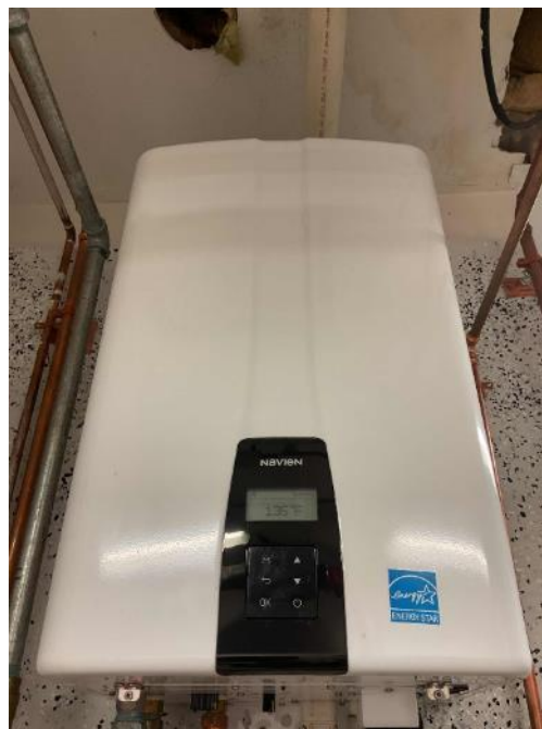
Navien Natural Gas Tankless Water Heater
