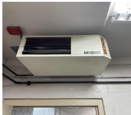
Reznor Gas-Fired Unit Heater
