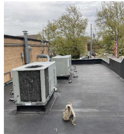
Flat Roof with Black Rubber Membrane
