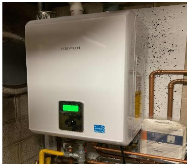
Navien Natural-Gas Tankless Water Heater
