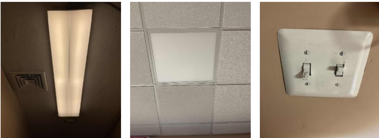
Typical Linear Fluorescent T8 and LED Light Panels with Wall Switches
