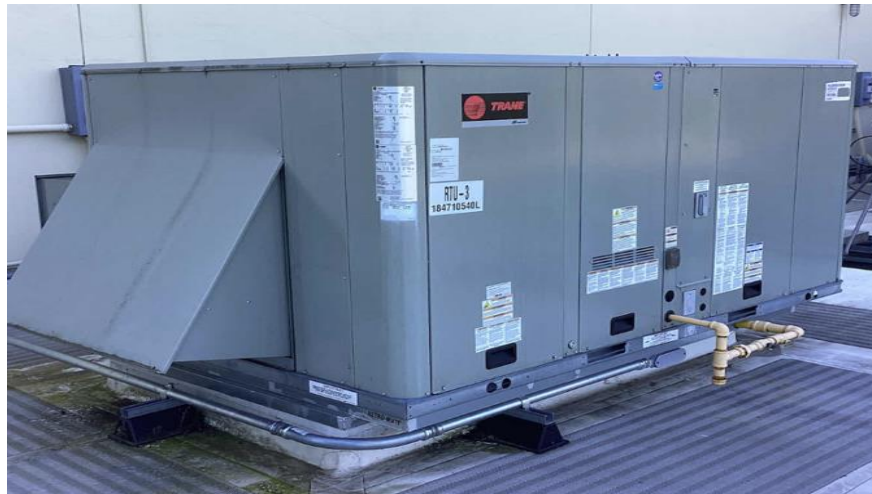
RTU on Roof
