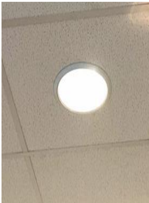
Recessed Halogen Lamps
