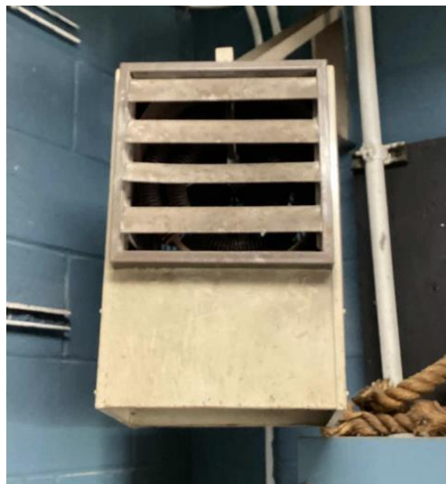
Electric Resistance Heater
