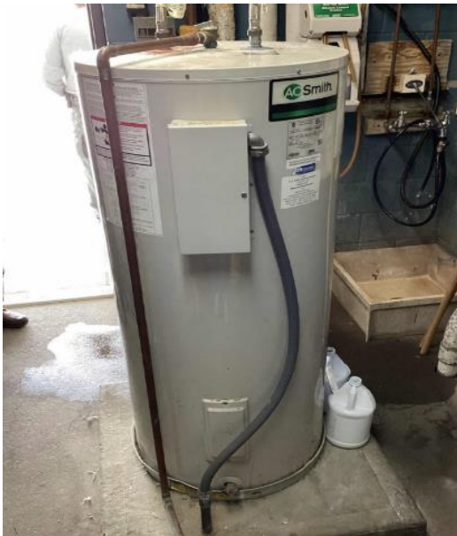
Storage Tank Water Heater
