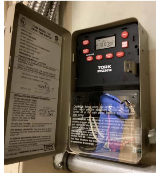
Timer for Exterior Building Lighting
