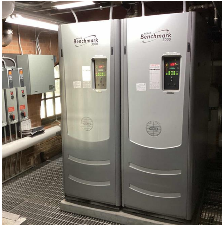
Condensing hot water boilers in CCRNJ Terminal
