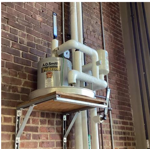
CCRNJ Terminal Electric Water Heater
