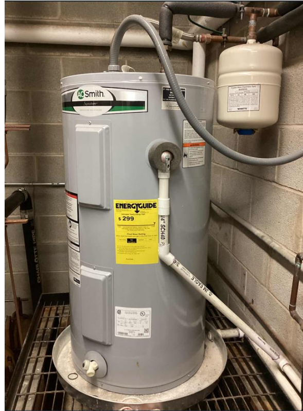
Electric DHW Tank
