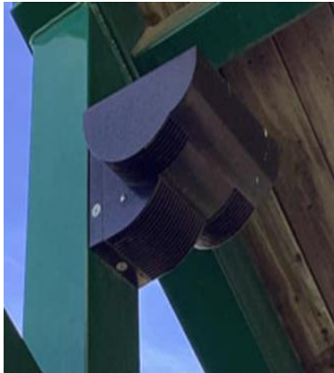
Metal Halide Lamps Under Pavilion
