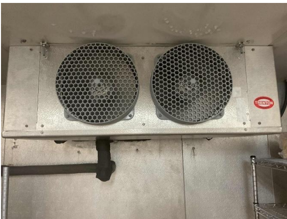
Walk-In Freezer Evaporator Unit
