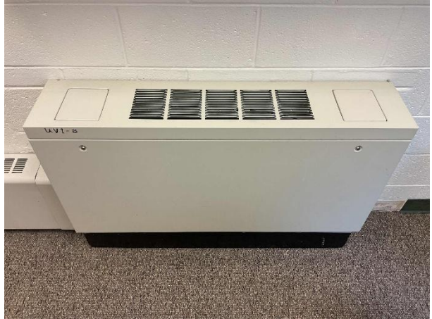
Typical Unit Ventilators in Offices & Band Room
