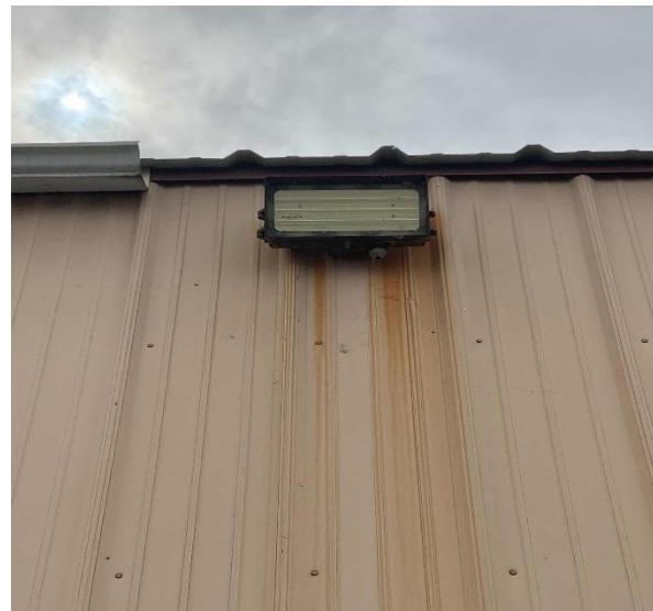
Left: Typical T8 Fixture Installed in Garages & Right: Typical Exterior LED Wall Pack Installed on Garages
