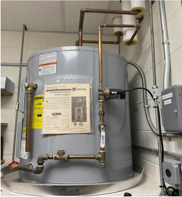
Electric Storage Water Heater Installed in Janitorial Closet
