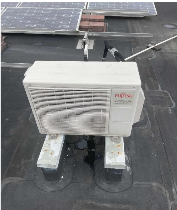
Typical Condensing Unit for Split System Air Sourced Units
