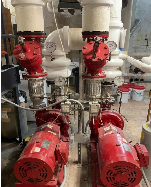
Heating Hot Water Pumps
