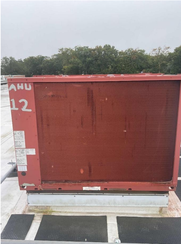
Typical TRANE RTU Mislabeled as AHU
