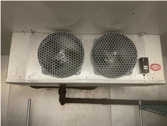
Walk-In Cooler Evaporator Unit
