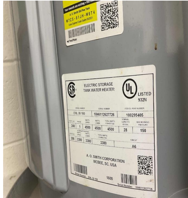
Electric Storage Water Heater Installed in Janitorial Closet
