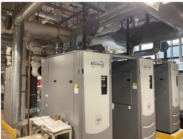
AERCO Benchmark Hot Water Boilers with Certification Information
