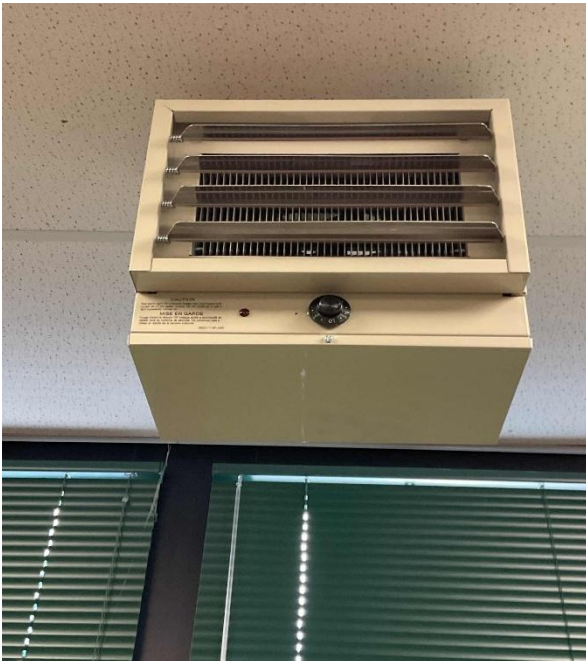
Typical Manually Controlled Electric Unit Heaters
