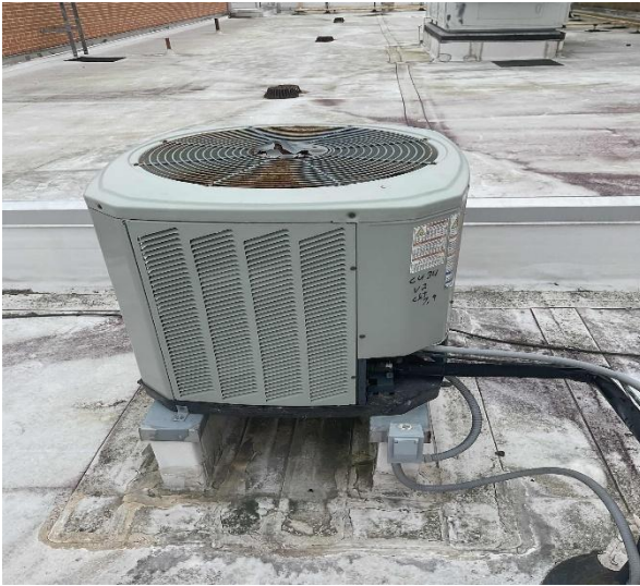
Typical Condensing Unit Utilized by Unit Ventilators
