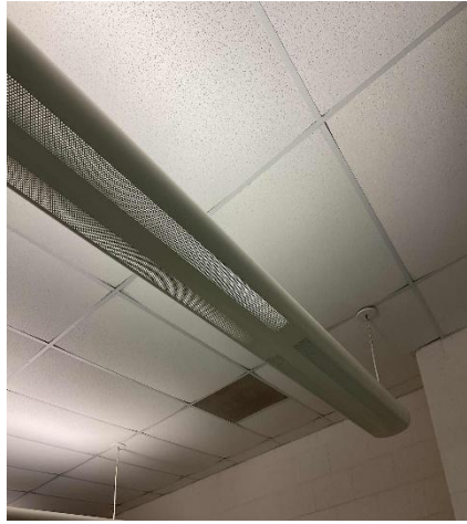
Typical Linear T8 & T8 U-Bend Linear Fluorescent Fixtures
