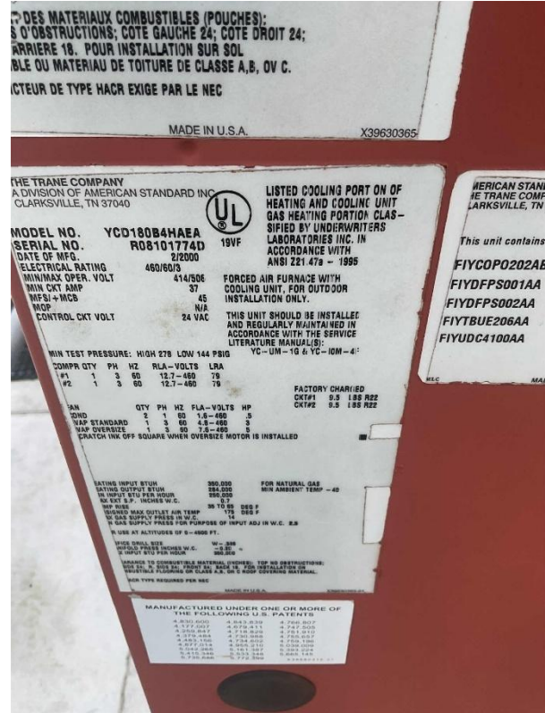
Typical TRANE RTU Mislabeled as AHU
