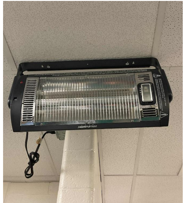
Typical Manually Controlled Electric Unit Heaters
