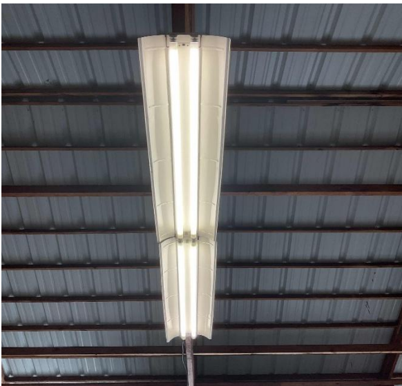
Left: Typical T8 Fixture Installed in Garages & Right: Typical Exterior LED Wall Pack Installed on Garages
