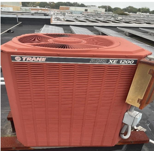
Typical Condensing Unit Utilized by Unit Ventilators
