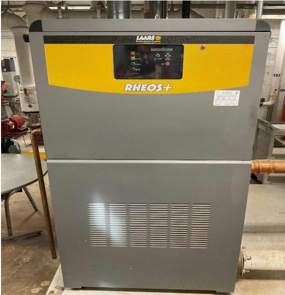
LAARS RHEOS+ Domestic Hot Water Boiler with Certification Information
