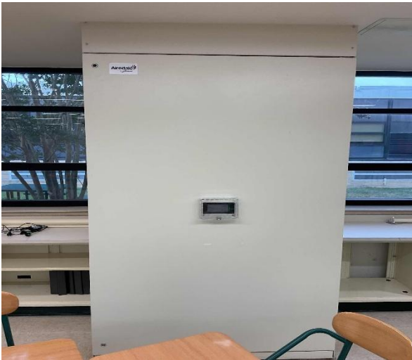
Typical AIREDALE Unit Ventilator
