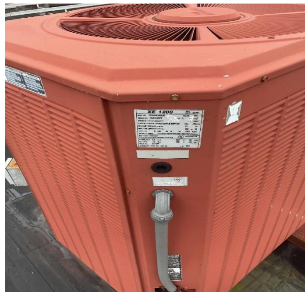
Typical Condensing Unit Utilized by Unit Ventilators
