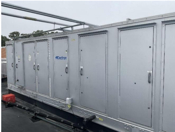
Dectron RTU Utilized for Dehumidification in Pool Room
