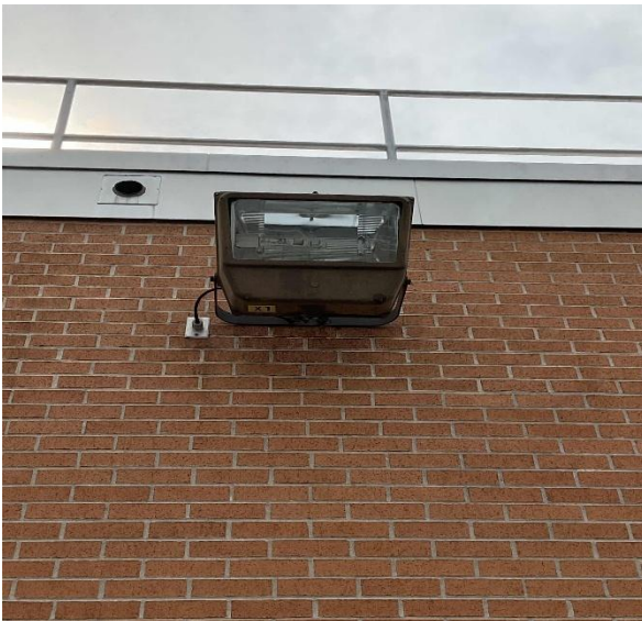
Left: Typical Metal Halide Wall Pack & Right: Typical LED Wall Pack
