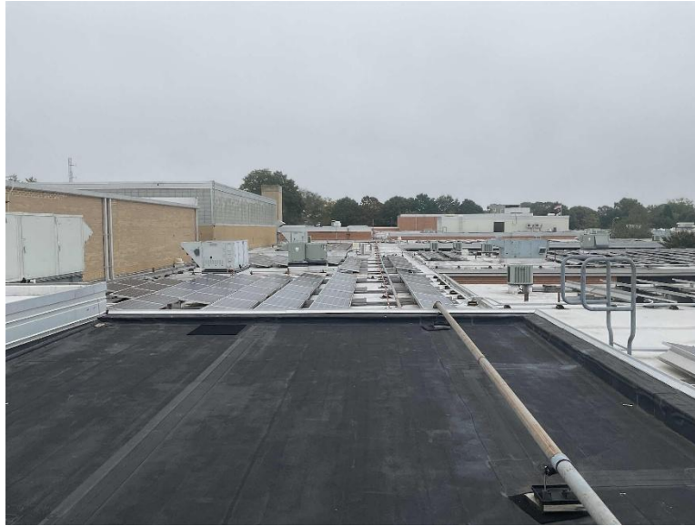
Flat Roof with Gray & Black Membrane
