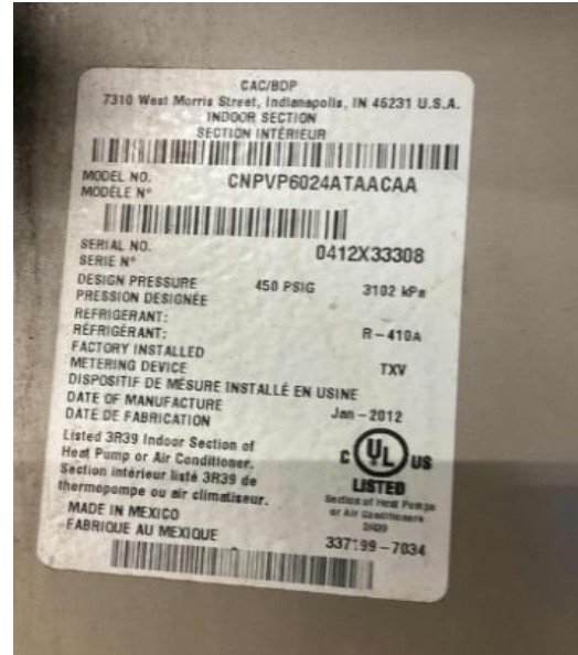
Indoor Evaporator Nameplate
