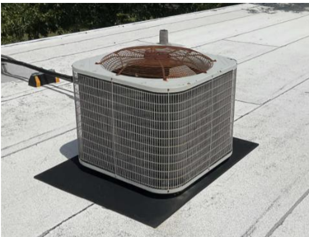
Front Office Exterior Condensing Unit
