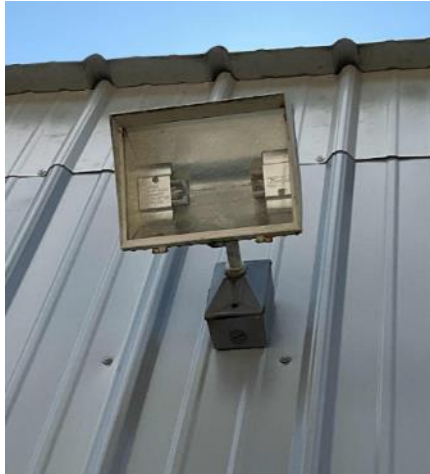
High Pressure Sodium Fixture
