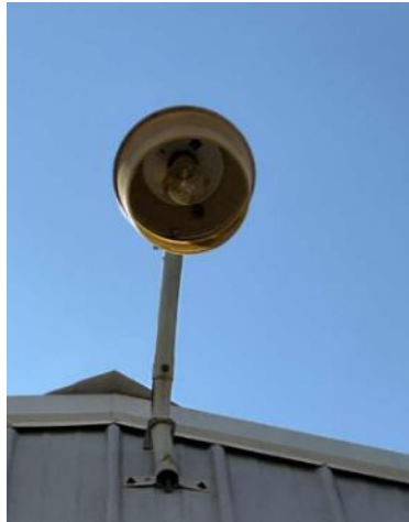
Metal Halide Fixture
