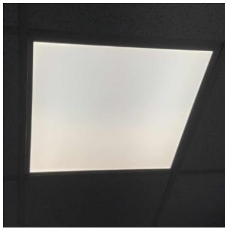
2-foot x 2-foot LED Fixture
