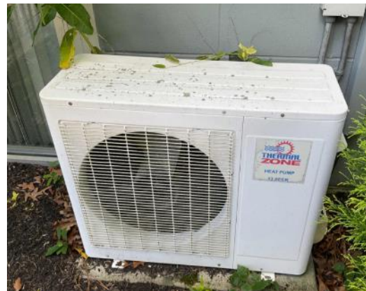
Ductless Mini-Split HP
