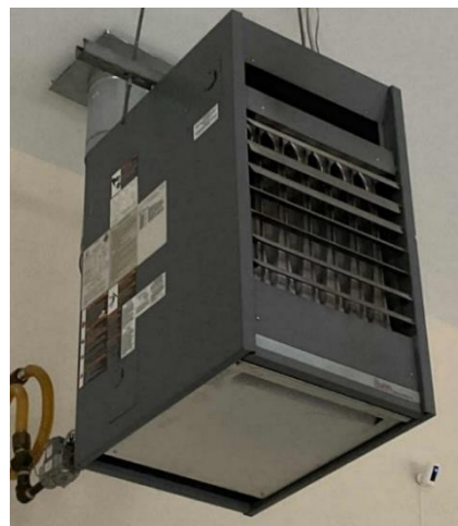
Gas Unit Heater in Garage
