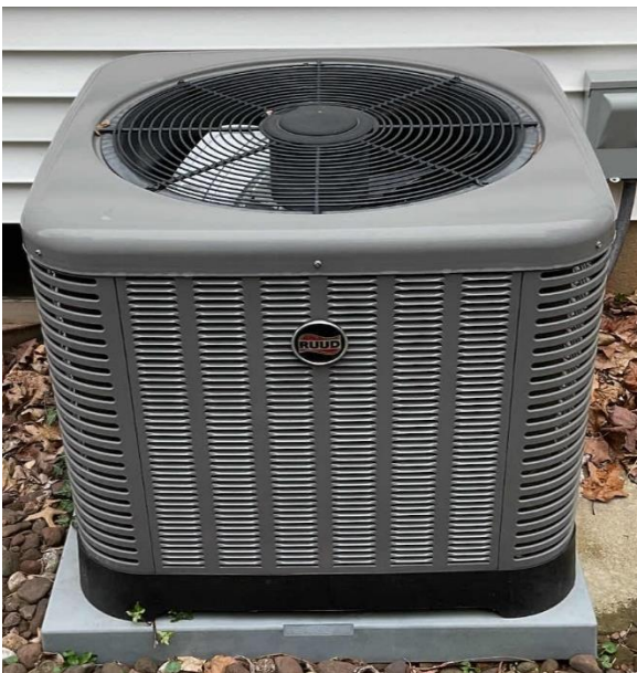
Rheem 3-ton Condenser Connected to AHU-2
