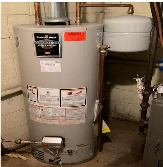
40-Gallon Gas Storage Tank Water Heater
