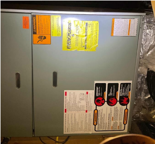
125 MBh Forced Air Furnace and AHU 1
