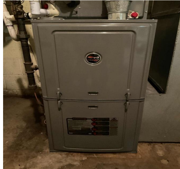
75 MBh Forced Air Furnace and AHU 2
