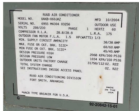
Ruud 5-ton Condenser Connected to AHU-1
