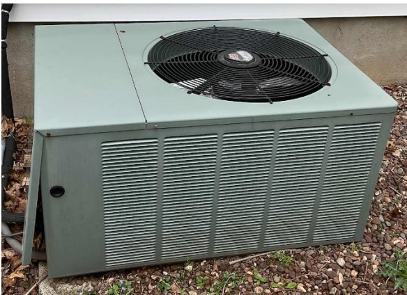
Ruud 5-ton Condenser Connected to AHU-1
