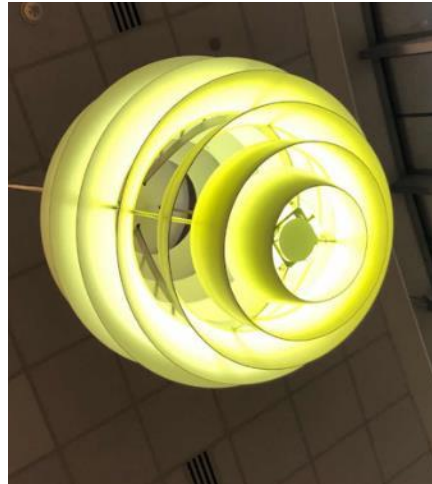
Metal Halide Fixture
