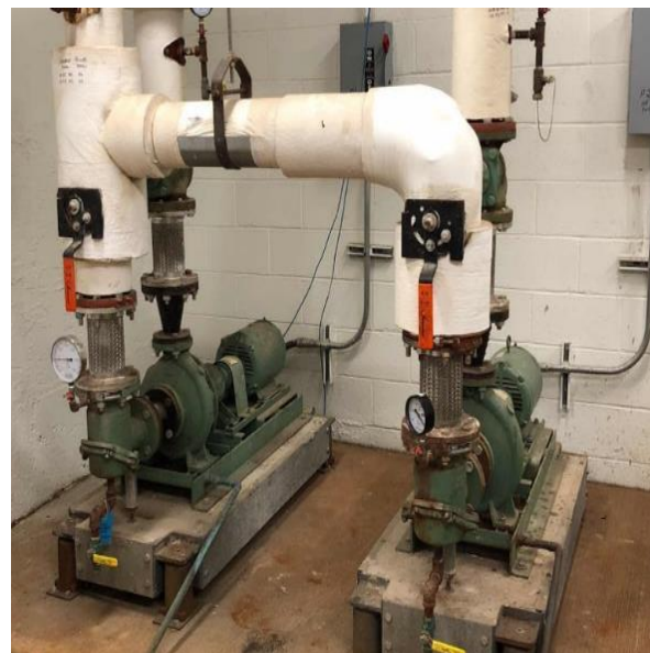
Heating Hot Water Pumps
