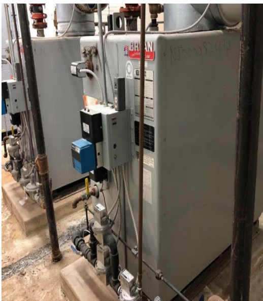
Heating Hot Water Boilers
