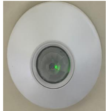
Wall Mounted Occupancy Sensor
