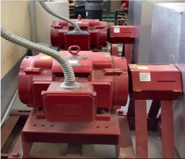
40 hp Variable Flow Condenser Water Pumps (P7 and P8)
