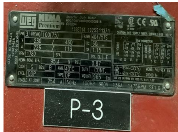
100 hp Geothermal Water Circulation Pumps
