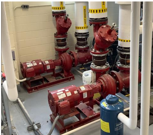
Hot Water Pumps - P5 and P6
