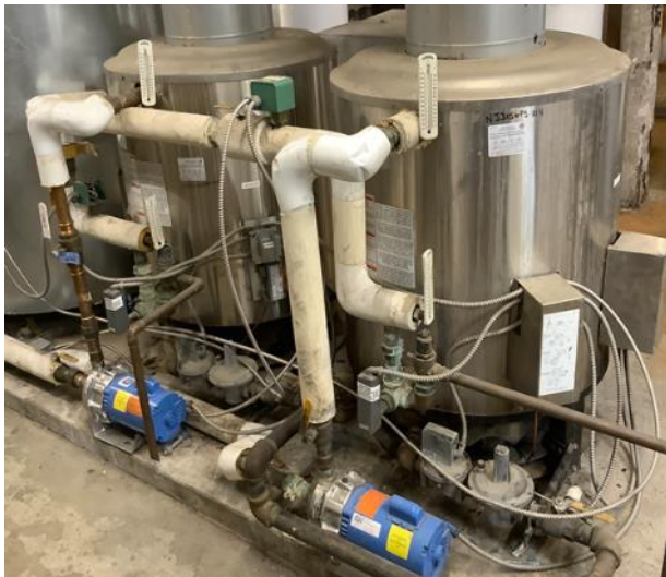
Domestic Hot Water (DHW) Boilers
