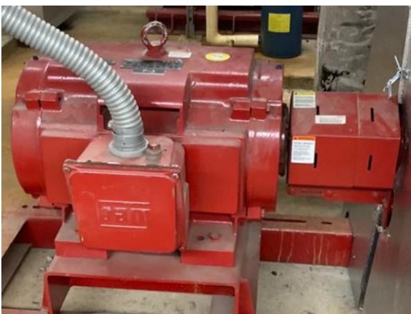
100 hp Geothermal Water Circulation Pumps
