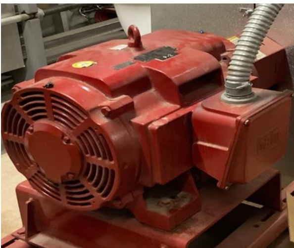
40 hp Variable Flow Condenser Water Pumps (P7 and P8)
