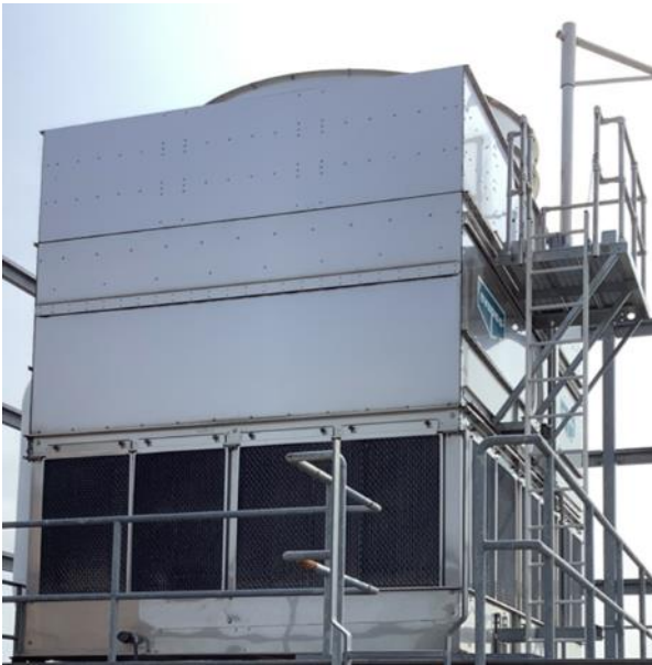
EVAPCO One-Cell Cooling Tower
