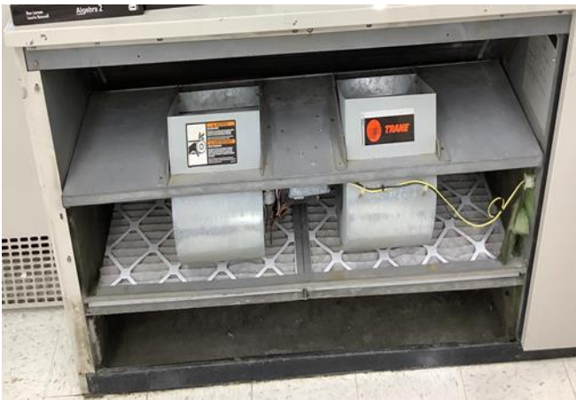
Trane Unit Ventilator WSHP
