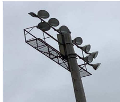
Pole Mounted Metal Halide Fixture
