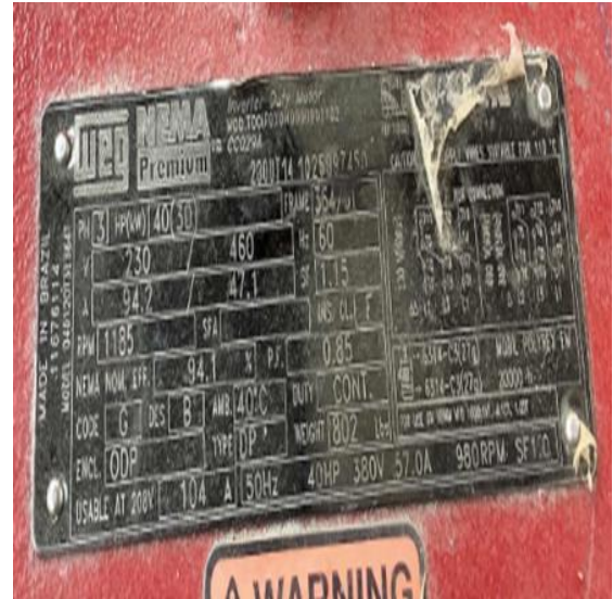
40 hp Variable Flow Condenser Water Pumps (P7 and P8)
