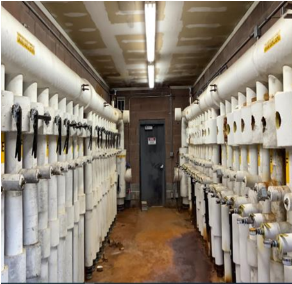
Geothermal System
