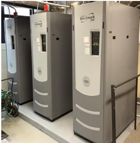
AERCO Condensing Boilers
