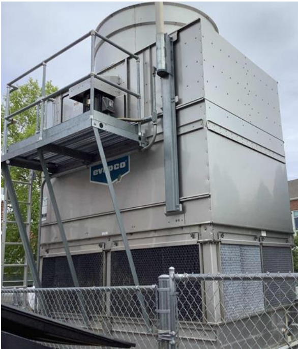
EVAPCO One Cell Cooling Tower
