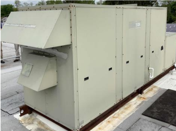
Packaged Water Source Heat Pump RTU-2
