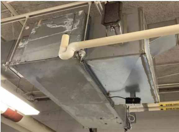
Typical Above Ceiling Mounted WSHP
