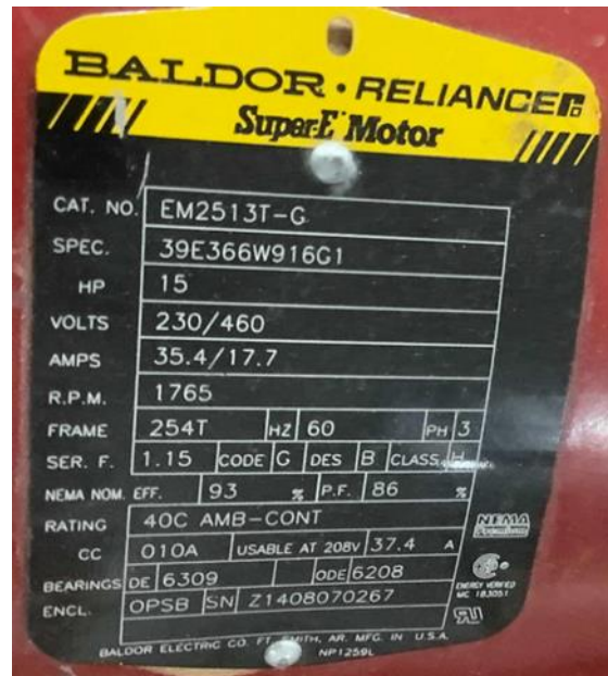
15 hp Variable Flow Condenser Water Pumps (P7 and P8)
