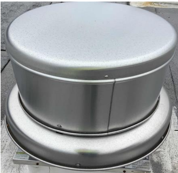
Typical Exhaust Air Fan
