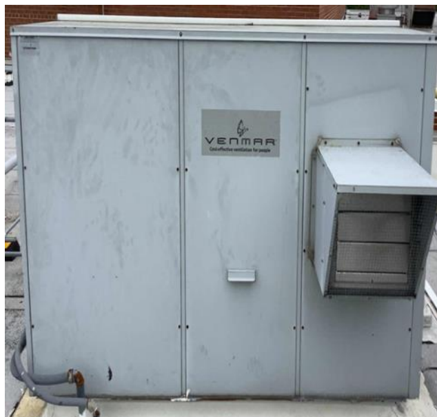
RTU-19 - ERV - Guidance Offices
