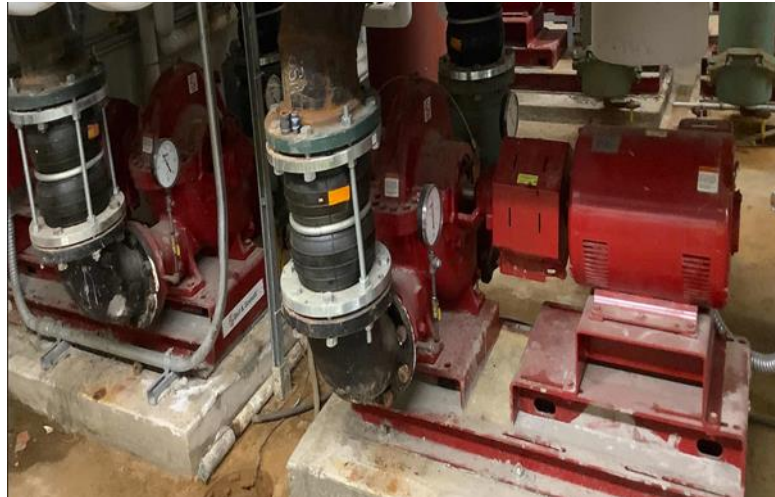
30 hp (P1 and P2) Field Water Circulation Pumps
