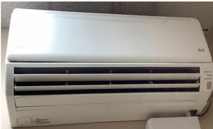
Indoor Evaporator (Heat Pump)
