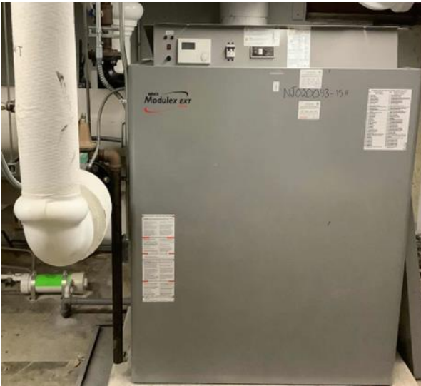
AERCO Condensing Hot Water Boiler
