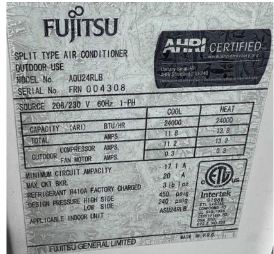
Ductless Air Source Heat Pump – Outdoor Condensing Unit
