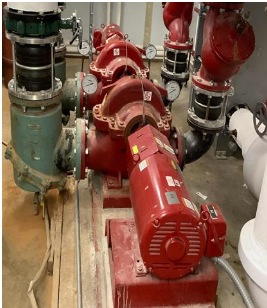
15 hp Variable Flow Condenser Water Pumps (P7 and P8)
