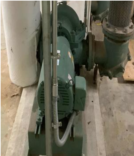
20 hp (P3 and P4) Water Circulation Pump
