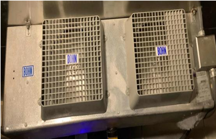
Evaporator - Walk-In Cooler
