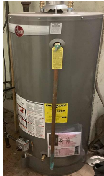
80-Gallon Gas Storage Tank Water Heater
