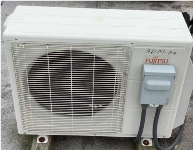
Ductless Air Source Heat Pump – Outdoor Condensing Unit
