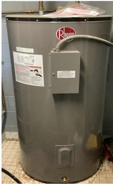
50-Gallon Electric Storage Tank Water Heater
