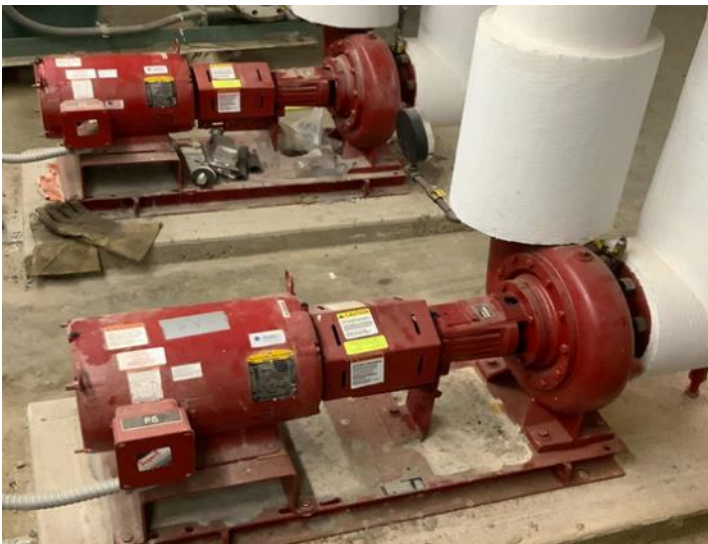
10 hp Variable Flow Hot Water Pumps (P5 and P6)
