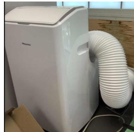
Indoor Evaporator (Portable AC)
