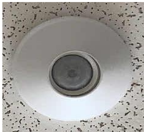
Ceiling Mounted Occupancy Sensor
