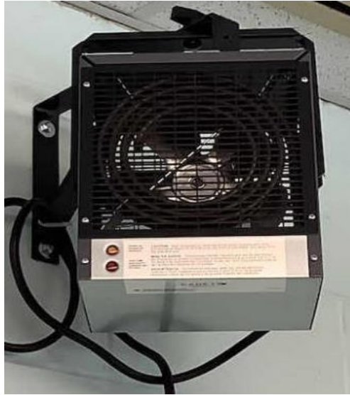
Ceiling Mounted Electric Resistance Heater
