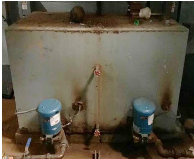
Boiler Condensate Pumps
