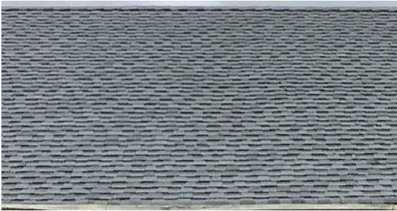
Asphalt Shingle Roof
