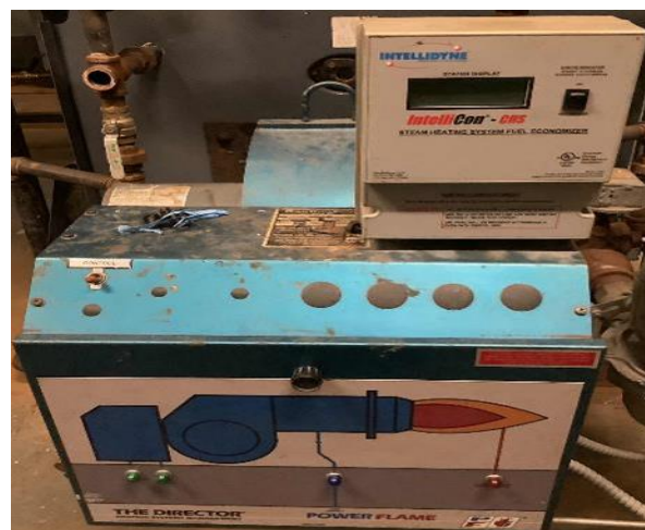
Forced Draft Combustion Fan and Burner Economizer
