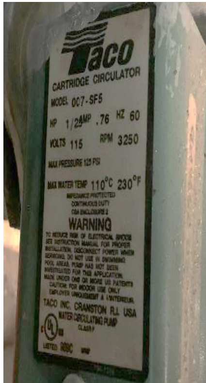
DHW Circulation Pump Name Plate
