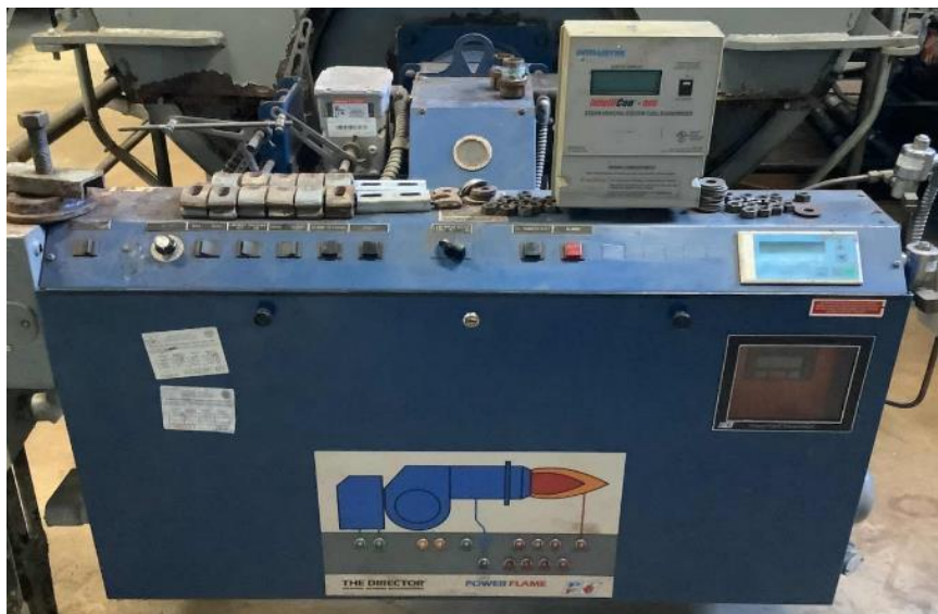
Forced Draft Combustion Fan and Burner Economizer
