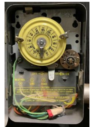
Time Clock for Exterior Lights
