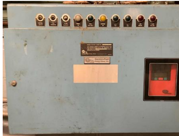
Boiler Control System
