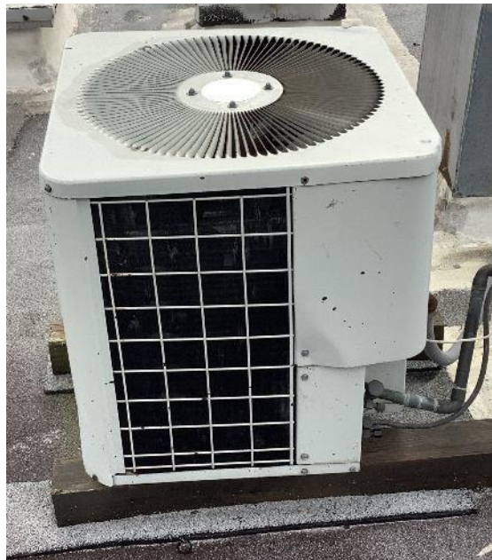
Split System AC Condensing Unit
