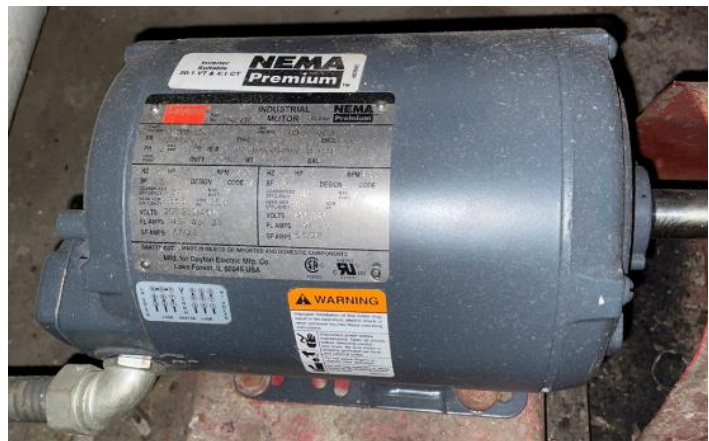
HHW Pump for Zone Distribution
