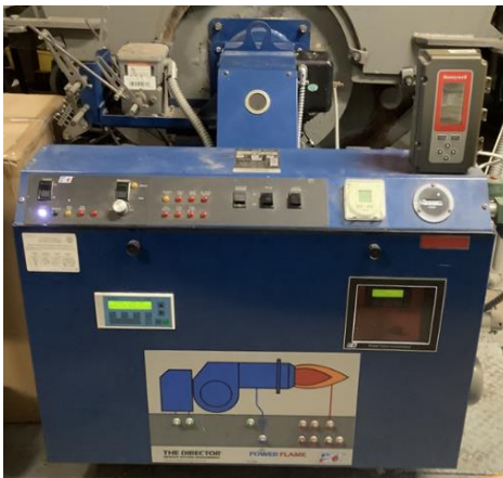
Boiler Burner
