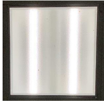
2-Foot T8 Equivalent LED Linear Tubes
