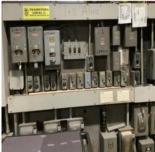
Heating Zone Control Panel
