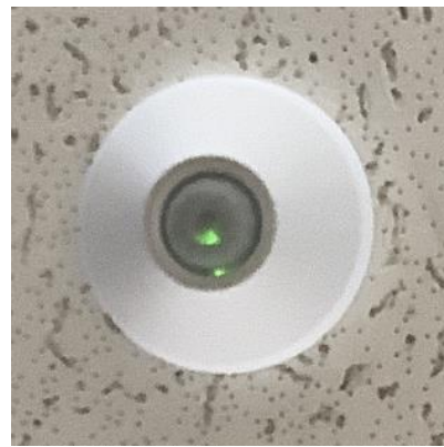
Ceiling Mounted Occupancy Sensor
