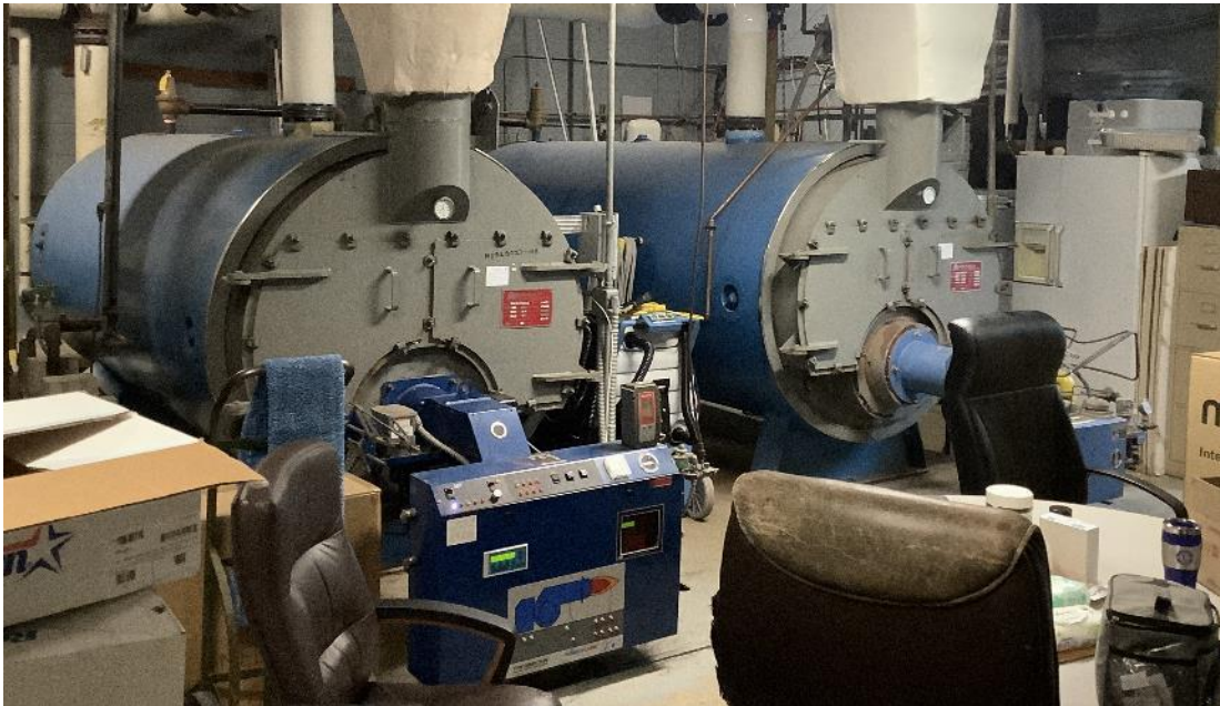
Non-Condensing Hot Water Boiler
