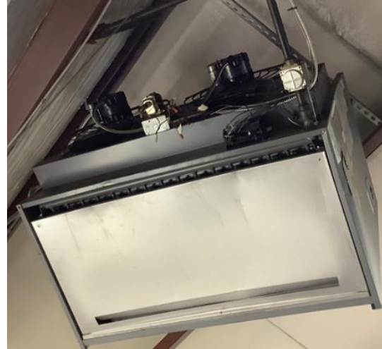
Gas-Fired Unit Heaters
