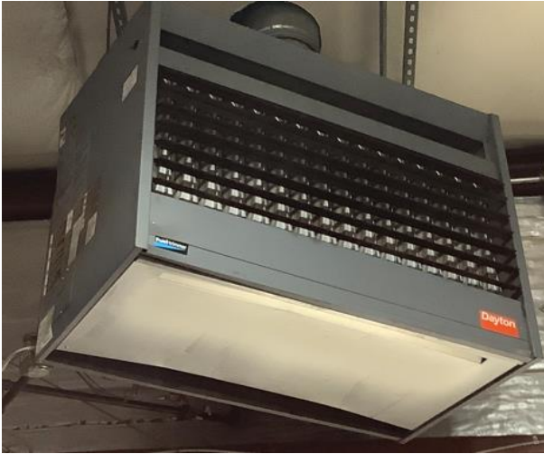
Gas-Fired Unit Heaters
