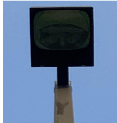
Metal Halide Fixture
