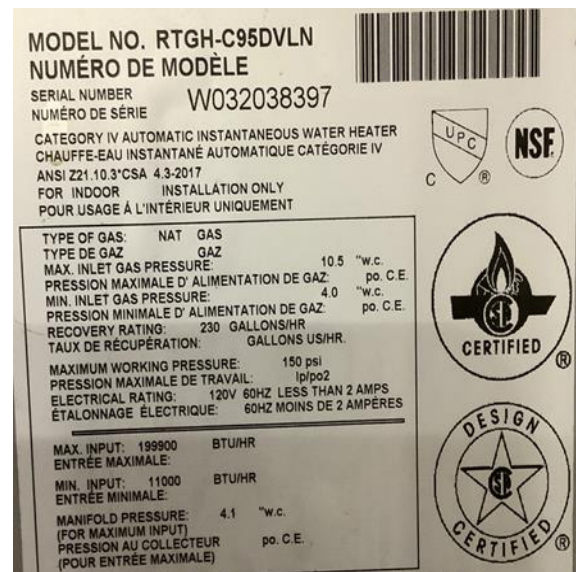
199.9 MBh Tankless Gas-Fired Water Heaters
