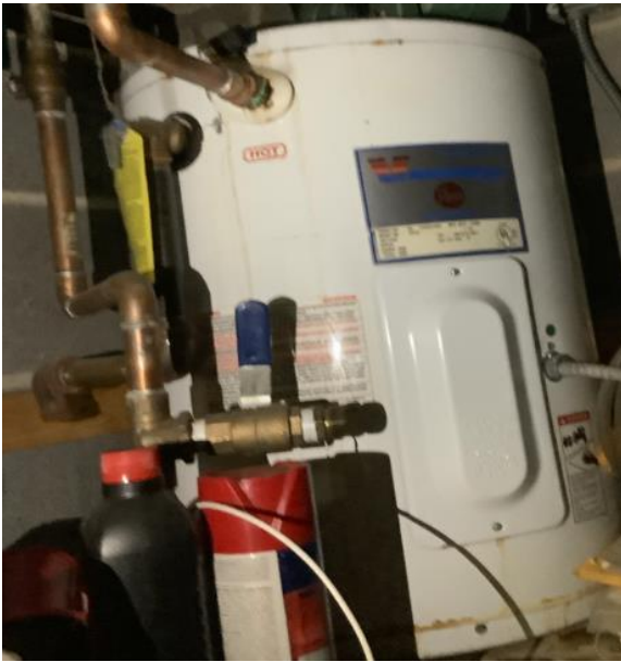
Electric Storage Tank Water Heater
