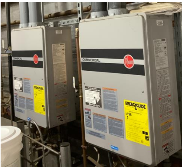
199.9 MBh Tankless Gas-Fired Water Heaters
