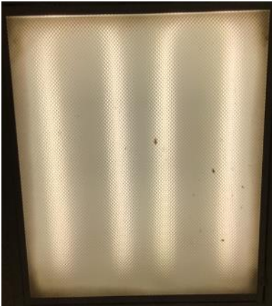
Linear T8 U-Bend Fixture
