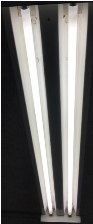
LED Tube Fixtures
