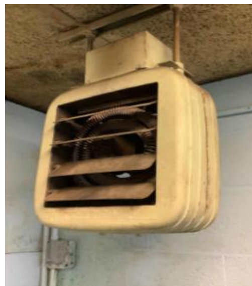
Electric Resistance Heater
